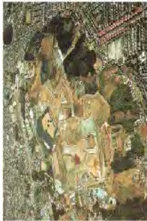
Shimmedai Disposal Site (~Mar. 2011)
