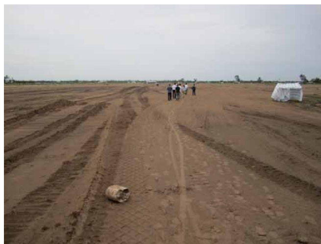
Photo 3.4.3 Song Hau 1 site (from south-west end of Power plant area)
