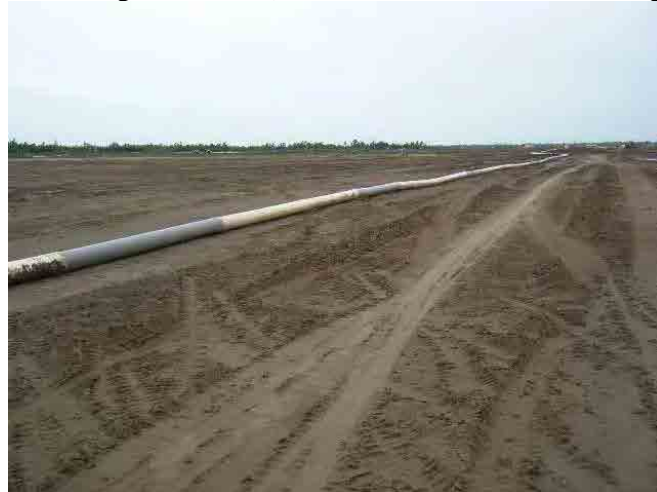
Photo 3.4.5 Steel pipe of Embankment material for Soil preparation work
