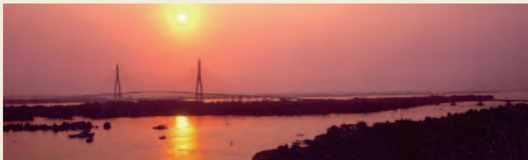
With the main bridge section extending 1,010 meters, the Can Tho Bridge is the longest cable-stayed bridge in Southeast Asia.
