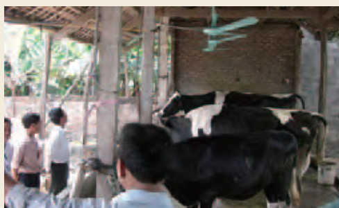
Cooling fans and anti-moisture devices were installed on the ceilings of cattle barns without walls as a heat management measure.
