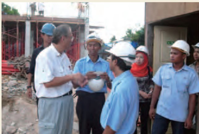
A Japanese expert providing guidance on earthquake-resistant design to local workers at the construction site.
