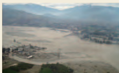
This bridge was washed away in the flooding. (Khyber Pakhtunkhwa Province)
