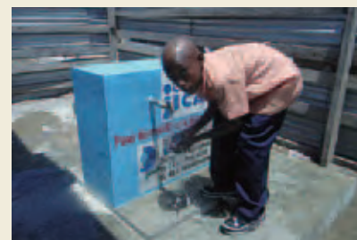
A public water hydrant established by the Project. From October 2010, cholera infections increased in Haiti, causing a large number of deaths. Efforts continue to deliver safe and clean water to the people of Haiti.
