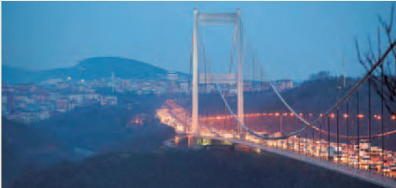
Large-scale bridges in Istanbul for which seismic reinforcement work has been completed.
