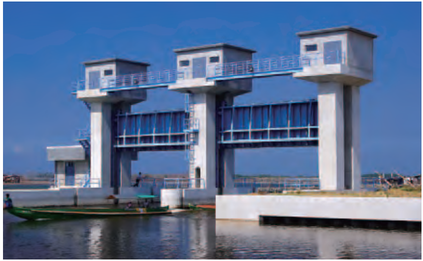
Lying on lowland terrain and susceptible to frequent flood damages, the Kamanava area in the Metro Manila, the Philippines, was installed with floodgate (photo) and drains, etc. by ODA Loans.
