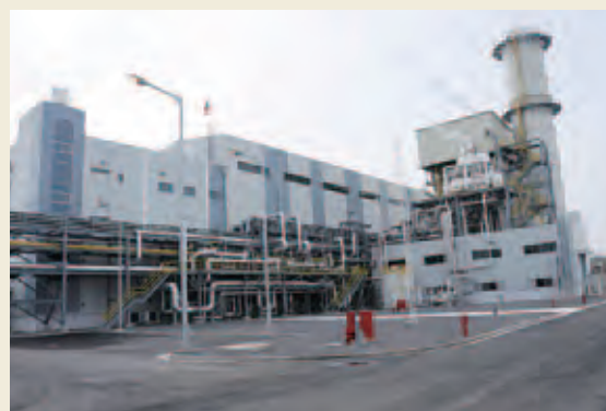
The completed Yerevan Combined Cycle Cogeneration Power Plant
