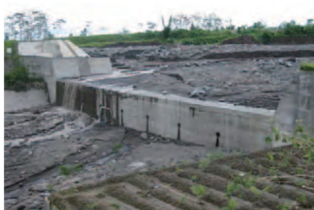
The sabo dam constructed with JICA cooperation preventing debris flow after the eruption of Mt. Merapi (Indonesia)
