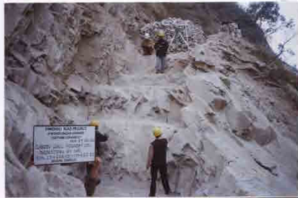
Photo No. 13 DATE : 29 December 2002 DESCRIPTION : Gabion Wall - Foundation Bedding Inspection by the Consultant LOCATION : Sta. 17+608-17+620
