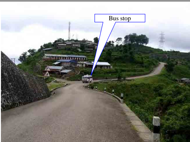
Traveling bus on the Sinduuli road (several times per day)
