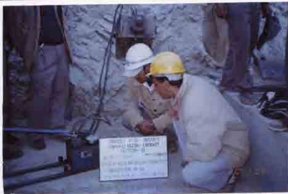
Photo No. 15 DATE : 20 January 2003 DESCRIPTION : Reinforced Earth Wall - B Anchor Pull Out Strength Test Inspection by the Consultant LOCATION : Sta. 17+529-17+533
