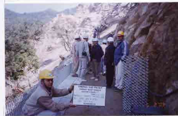
Photo No. 16 DATE : 05 February 2003 DESCRIPTION : Monthly Safety Patrolling by DOR, NK and HT-JV LOCATION : Sta. 17+500
