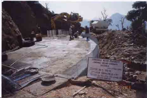
Photo No. 16 DATE : 09 January 2003 DESCRIPTION : Reinforced Earth Wall - B 3rd Layer Compaction by 1 ton Roller LOCATION : Sta. 13+048-13+072
