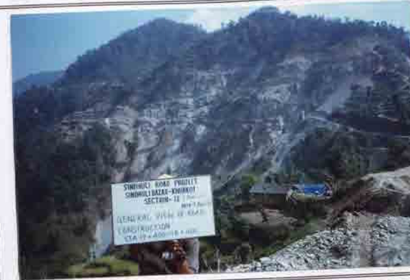
Photo No. 4 DATE : 19 November 2002 DESCRIPTION : General View of Road Construction LOCATION : Sta. 17+400-18+400
