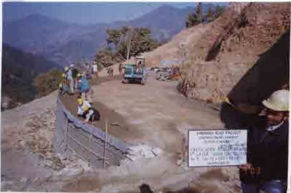
Photo No. 17 DATE : 20 January 2003 DESCRIPTION : Reinforced Earth Wall - B 7th Layer Construction LOCATION : Sta. 13+048-13+072
