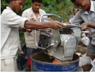
Photo 9: Compaction Layers by Monkey Jumper
