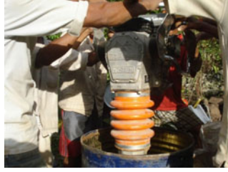
Photo 9: Compaction Layers by Monkey Jumper
