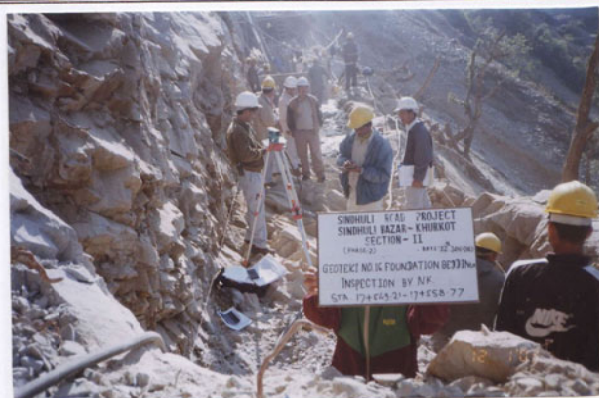
Photo No. 14 DATE : 12 January 2003 DESCRIPTION : Reinforced Earth Wall - B Foundation Bedding Inspection by the Consultant LOCATION : Sta. 17+549-17+558
