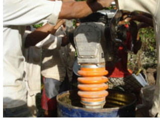
Photo 9: Compaction Layers by Monkey Jumper
