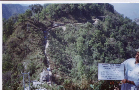
Photo No. 12 DATE : 18 April 2003 DESCRIPTION : General View of Road Construction LOCATION : Sta. 19+300-19+000
