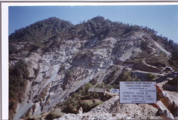
Photo No. 7 DATE : 20 January 2003 DESCRIPTION : General View of Road Construction LOCATION : Sta. 17+400~18+300
