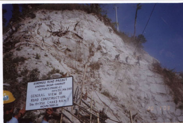
Photo No. 9 DATE : 20 January 2003 DESCRIPTION : General View of Road Construction LOCATION : Sta. 19+950
