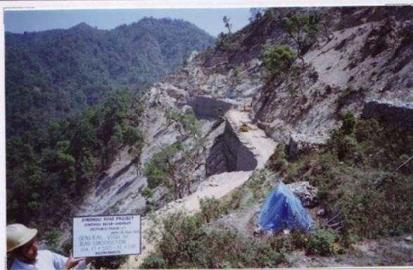
Photo No. 11 DATE : 18 April 2003 DESCRIPTION : General View of Road Construction LOCATION : Sta. 17+500-17+700
