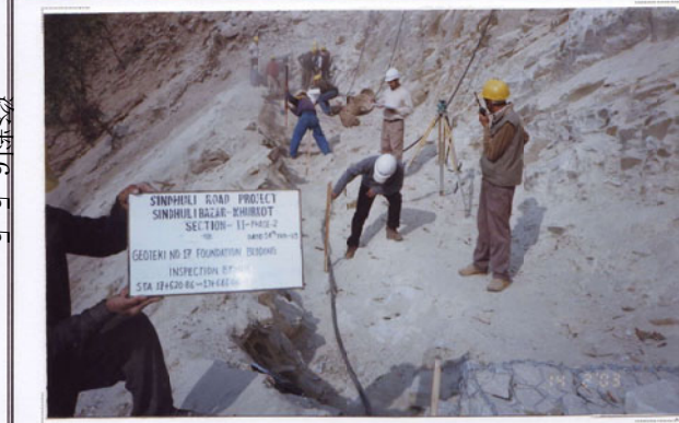
Photo No. 14 DATE : 14 February 2003 DESCRIPTION : Reinforced Earth Wall Foundation Inspection by the Consultant LOCATION : Sta. 17+620-17+646
