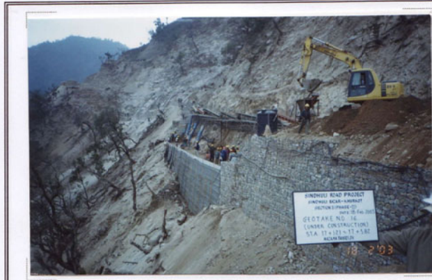
Photo No. 13 DATE : 18 February 2003 DESCRIPTION : Construction of Reinforced Earth Wall LOCATION : Sta. 17+521-17+582
