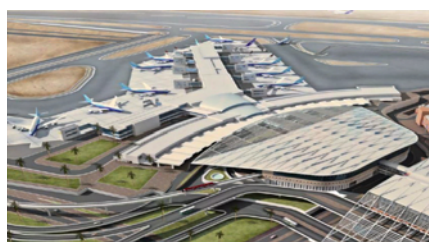
Image – Terminal 2 Renovation
