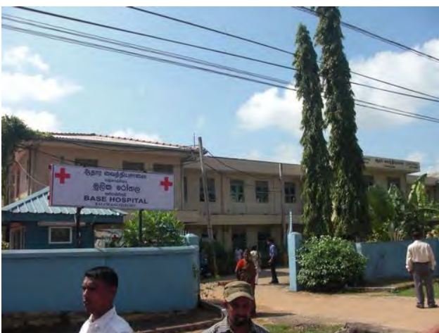
Front view of the Hospital
