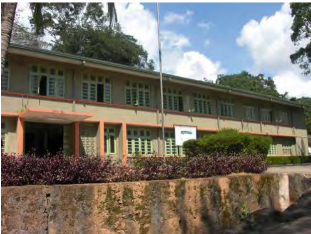
Front view of the Hospital
