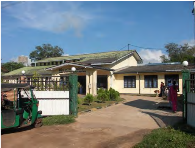
Front view of the Hospital
