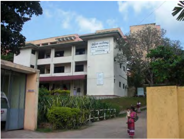
Front view of the Hospital
