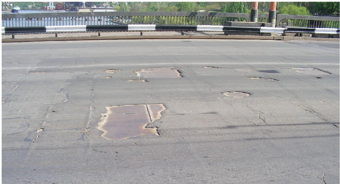
Figure 8.3.11 Surfacing on the steel deck of Ingul bridge in Mykolaiv
