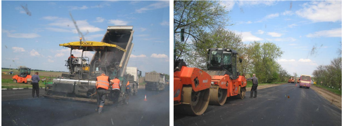
Figure 8.3.5 Maintenance work between Mykolaiv and Odessa on M14, May 2011.
