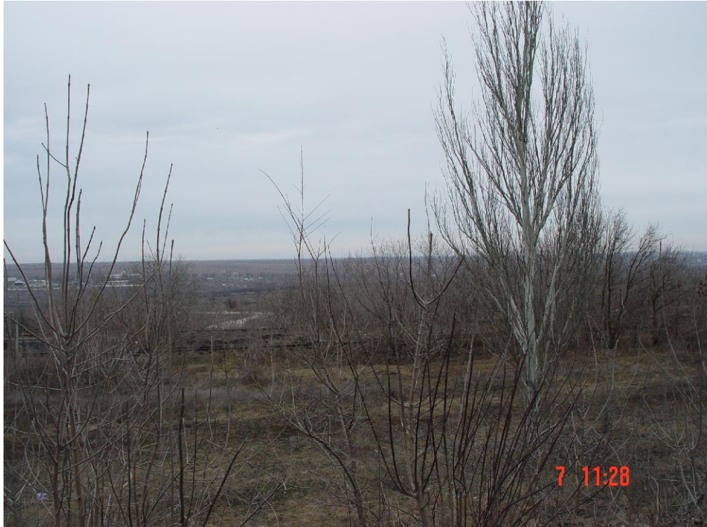
Figure 6.1.11 The Embankment on the Interchange “Clover Leaf”
