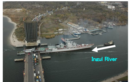
② Ingul Bridge(Navigation Open time)
