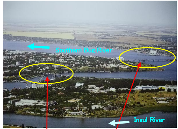
① Ingul Bridge, Vavarovsky Bridge
