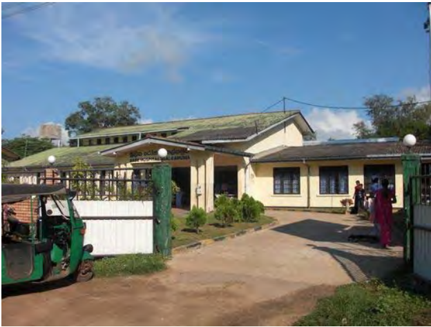
Front view of the Hospital
