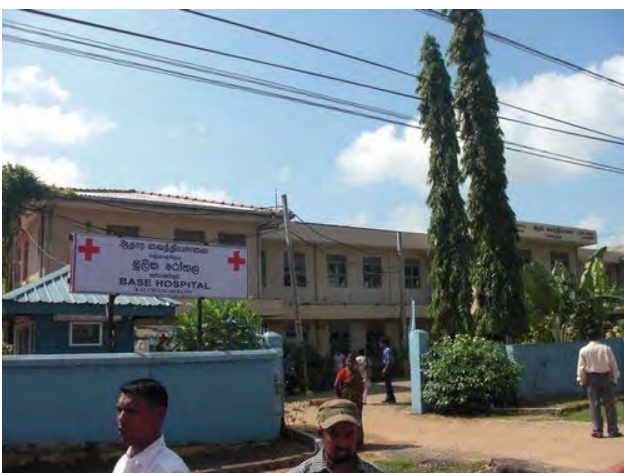
Front view of the Hospital
