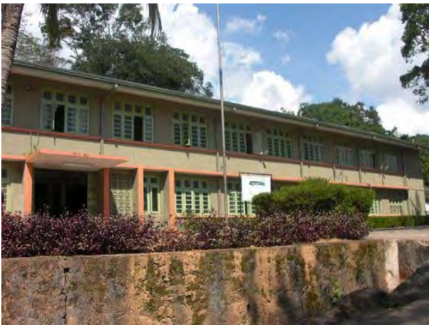
Front view of the Hospital
