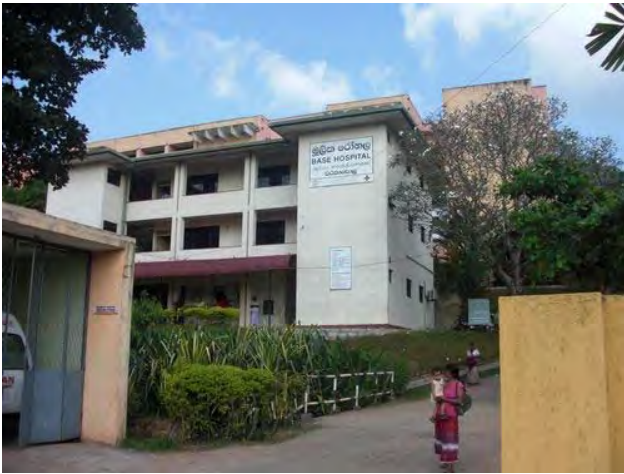
Front view of the Hospital
