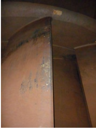
Photo-3 Paint on Stay Ring and Stay Vane
