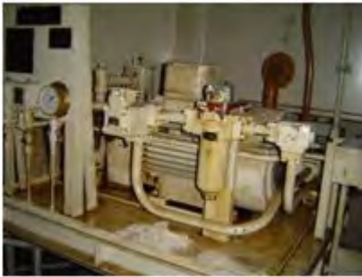
Photo 3.1-9 Oil-gathering around oil lift pump
