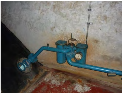
Photo-28 Filter for Shaft Seal Supply Water
