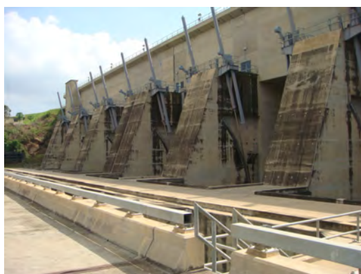
Photo 3.5-6 Main Spillway from downstream
