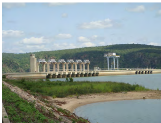
Photo 3.5-1 View of main structures from upstream
