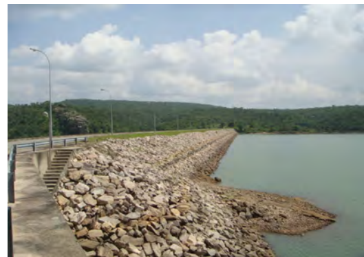
Photo 3.5-2 View of rock-fill dam
