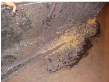
Photo-1 Repair welded at Flipper on Draft Tube Core
