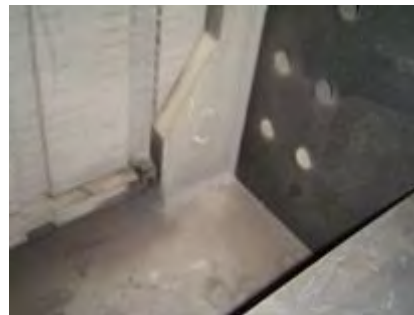
Photo 3.1-5 Present condition of rotor spider (2G2)
