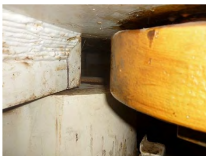
Photo-22 Stopper of Regulation Ring
