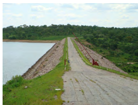
Photo 3.5-3 Saddle dam from right abutment
