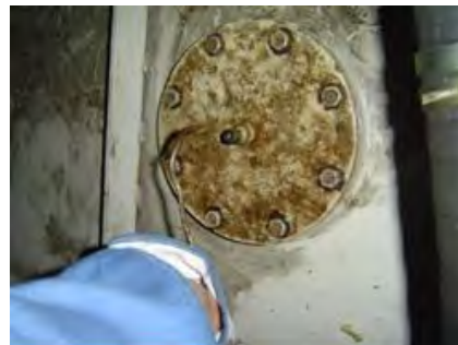
Photo 3.1-15 Oil temperature sensor
