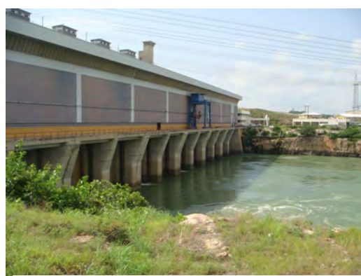
Photo 3.5-4 Powerhouse and tailrace afterbay
