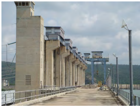
Photo 3.5-5 Intake and Gantry Crane
