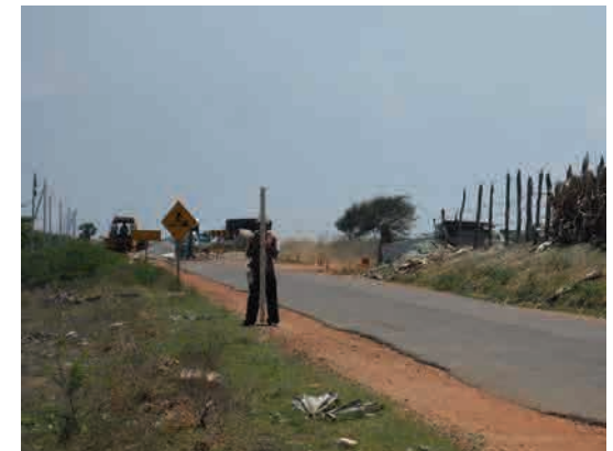
Photo Control Point Survey (Leveling)
