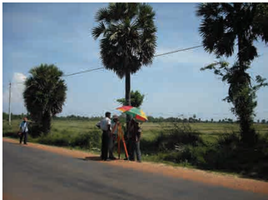
Photo Control Point Survey (Leveling)
