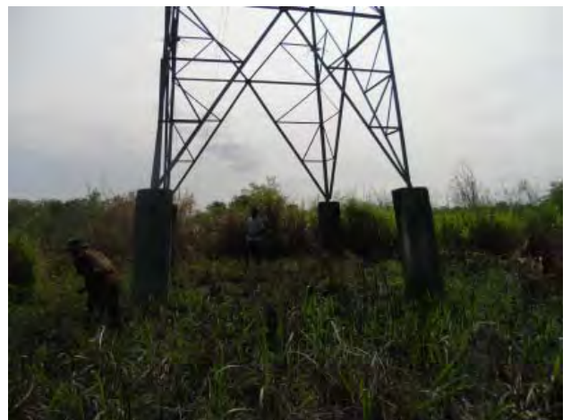
Tower Foundation at the East Bank of the Erap River
