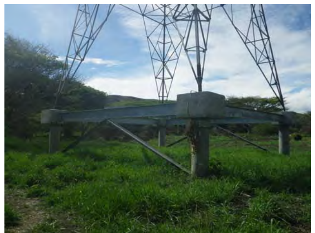
Bent Pile Foundation
