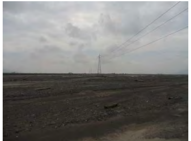
Transmission Line Crossing over the Markham River
