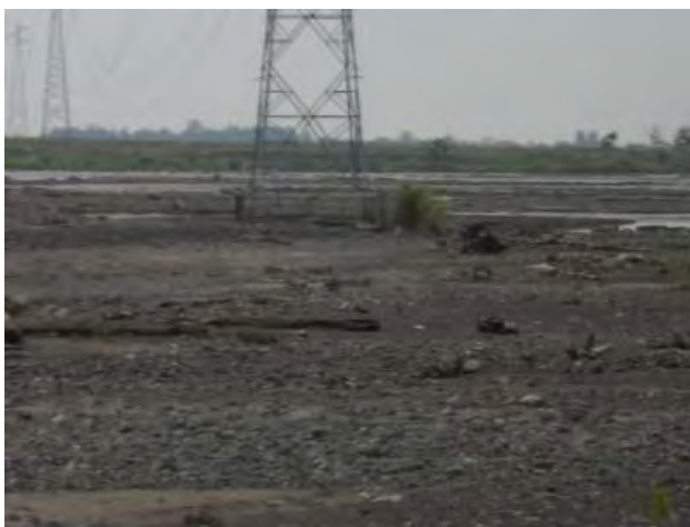
Tower Foundation in Markham River
