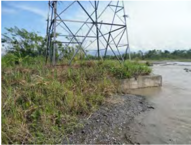
Tower Foundation at the Middle Bank of the Erap River
