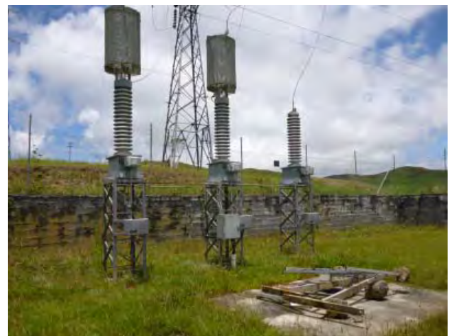
Line Trap and Potential Device
