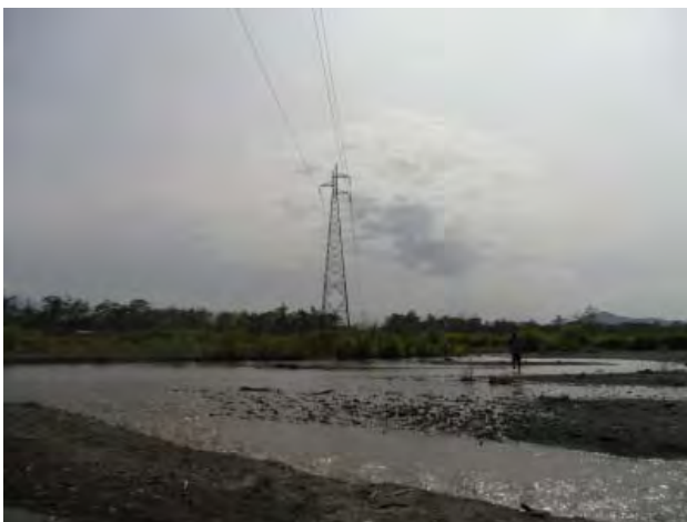
Transmission Line Crossing over the Erap River
