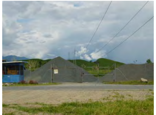
Rock Yard near Planned Singsing Substation Site
