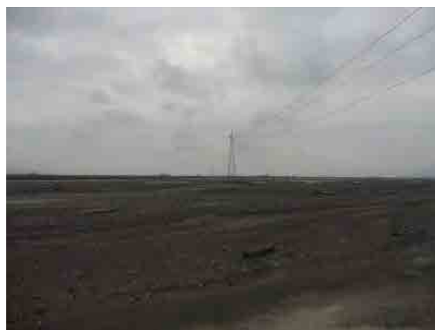
Transmission Line Crossing over the Markham River
