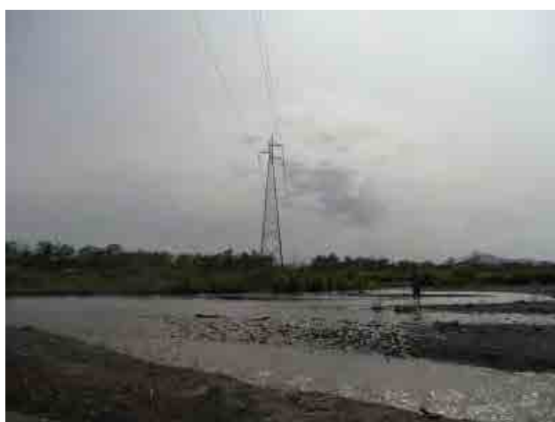
Transmission Line Crossing over the Erap River
