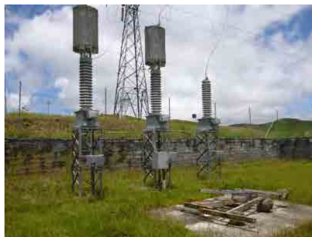
Line Trap and Potential Device
