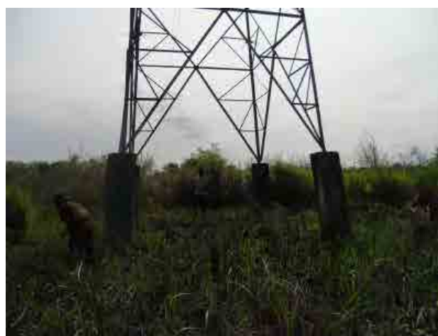
Tower Foundation at the East Bank of the Erap River
