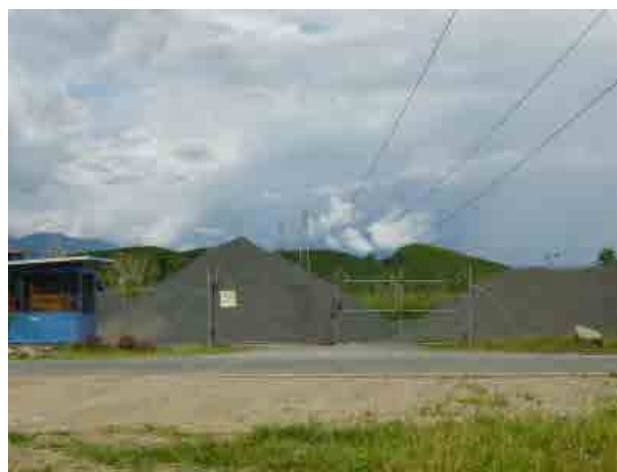
Rock Yard near Planned Singsing Substation Site
