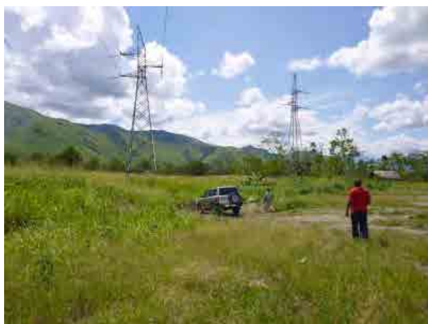
Planned Singsing Substation Site (2/2)
