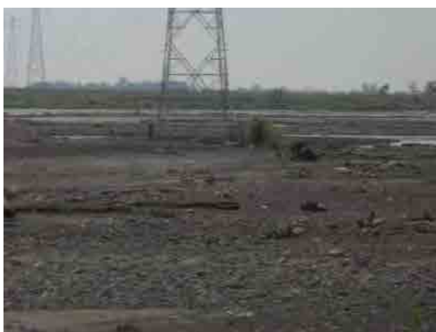
Tower Foundation in Markham River
