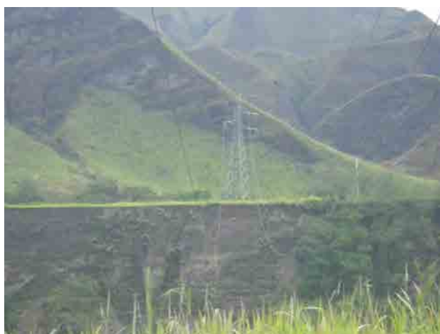
Transmission Line Crossing over the Leron River (2/2)
