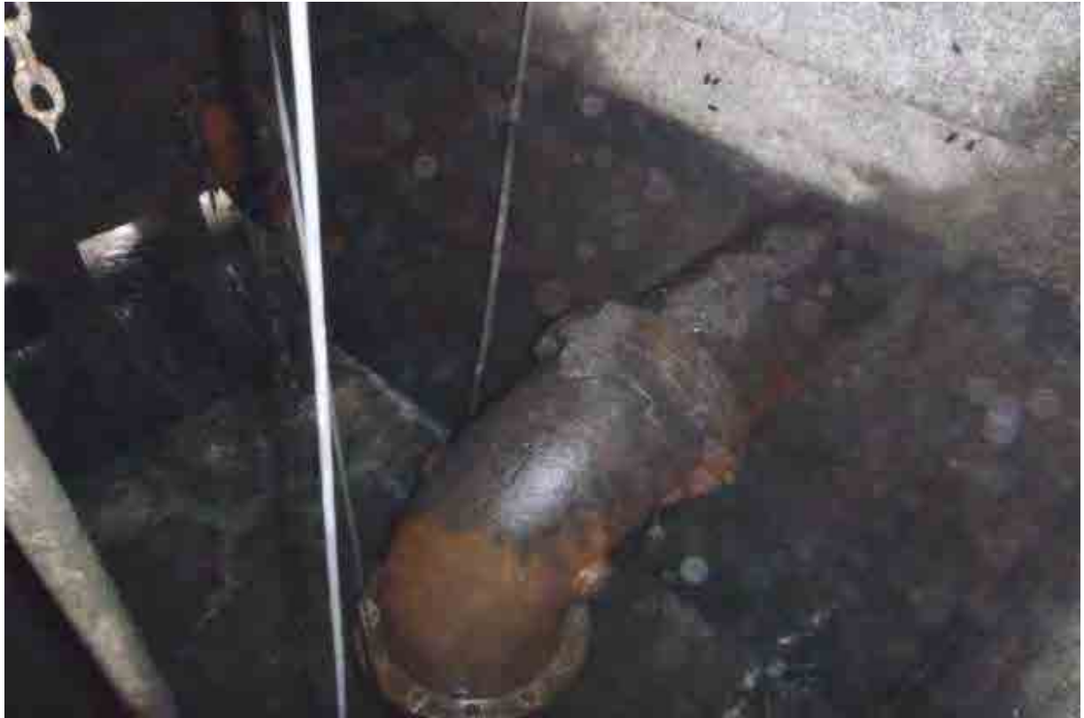
1k. Corrosion Condition; medium level of corrosion
