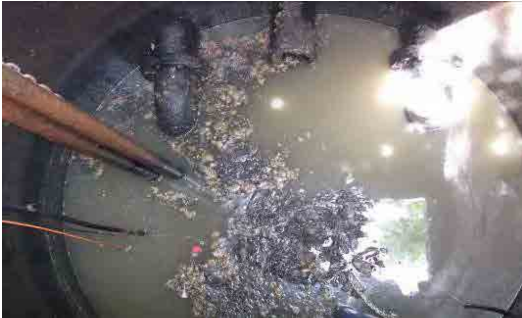
1a. Pump pit leakage Condition; there could be leakages below, middle pipe is spare pipe. Corrosion condition; Corrosion is occurring on steel pipes.
