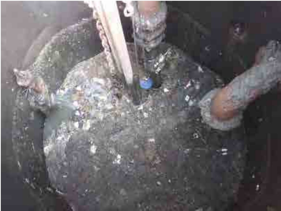
1c: Steel Rod Exposed; Most Steel Pressure Pipes are rusting
