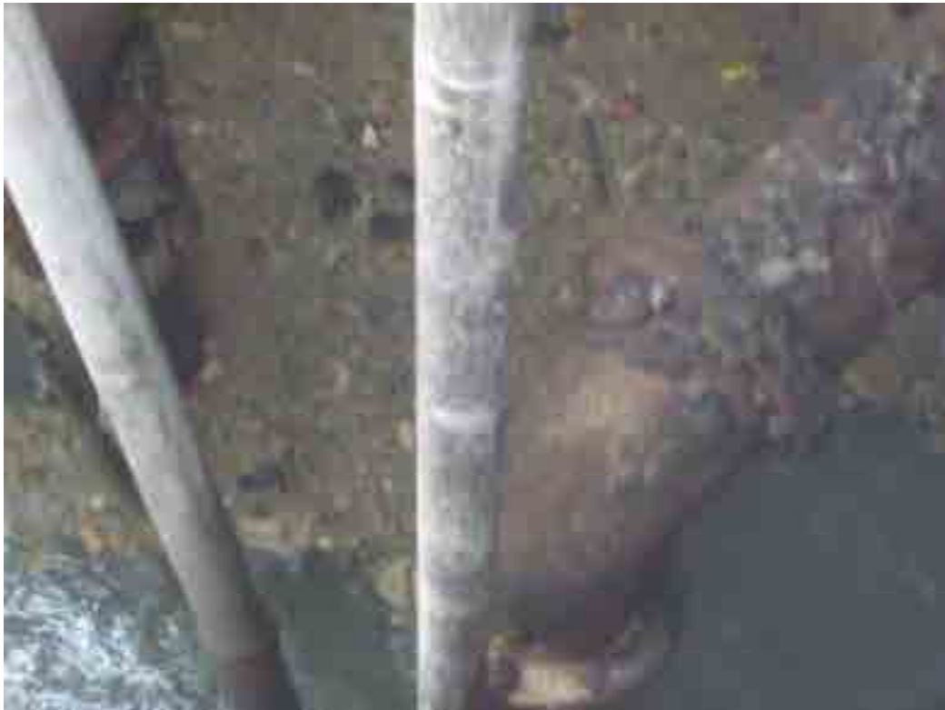
1e. Pressure Pipes are corroding like this one.
