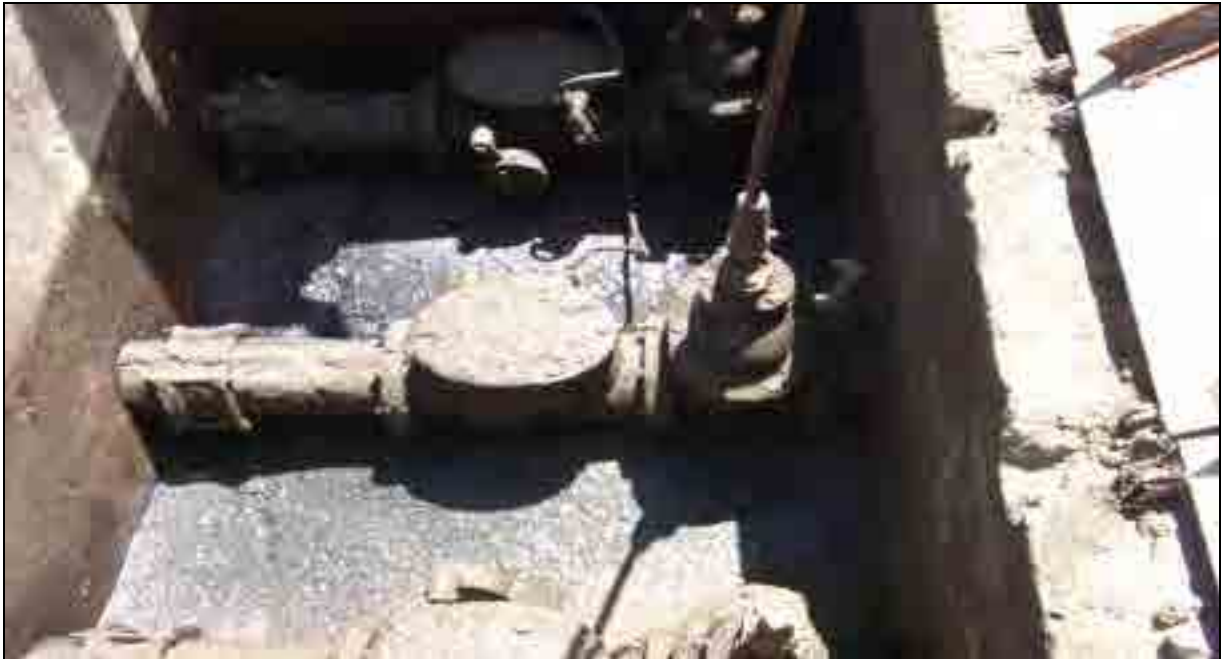
2b. Corrosion condition; medium level of corrosion occurring on steel
