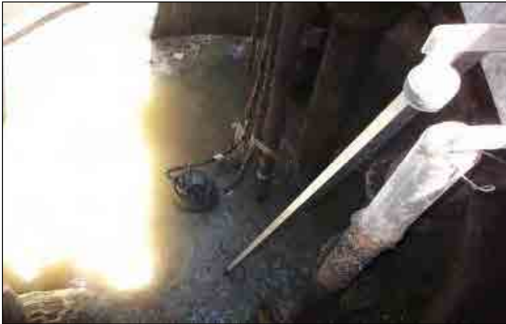
1b. Pump Pit Leakage Condition; Not many leakages
