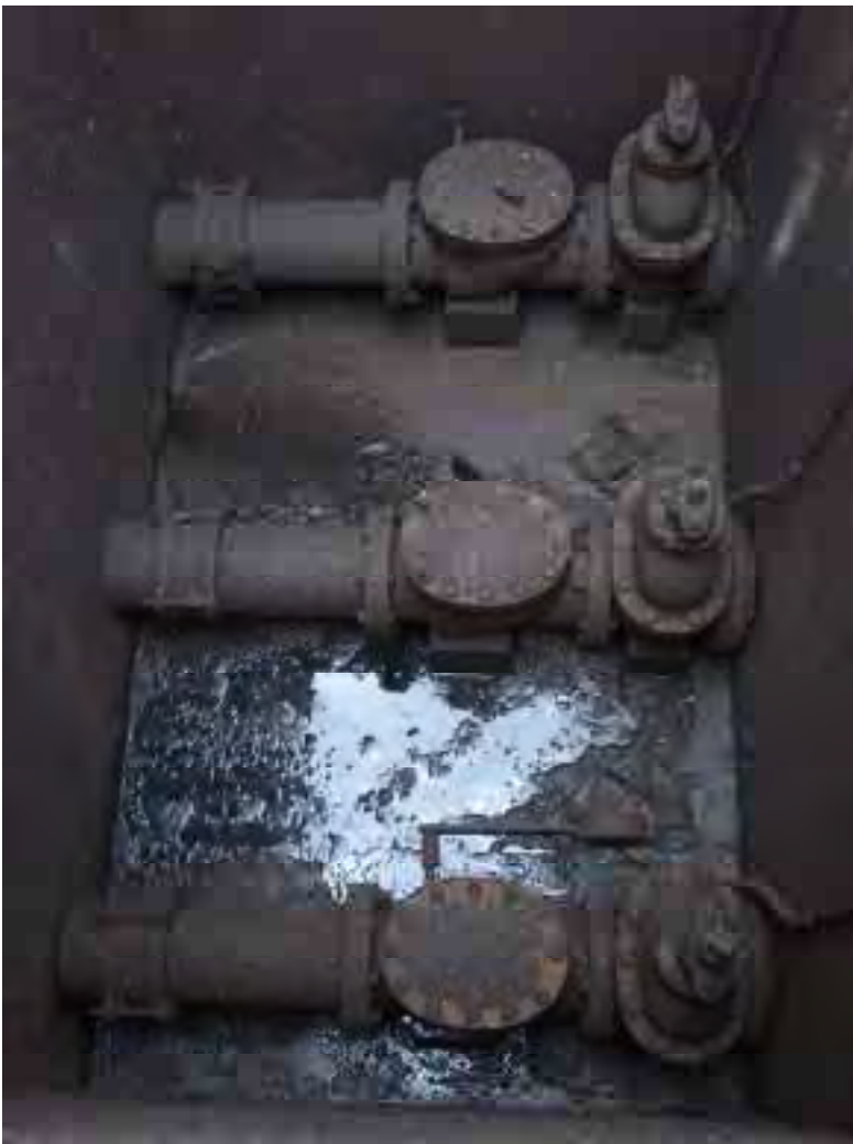
2b. Exposure of Steel and Corrosion
