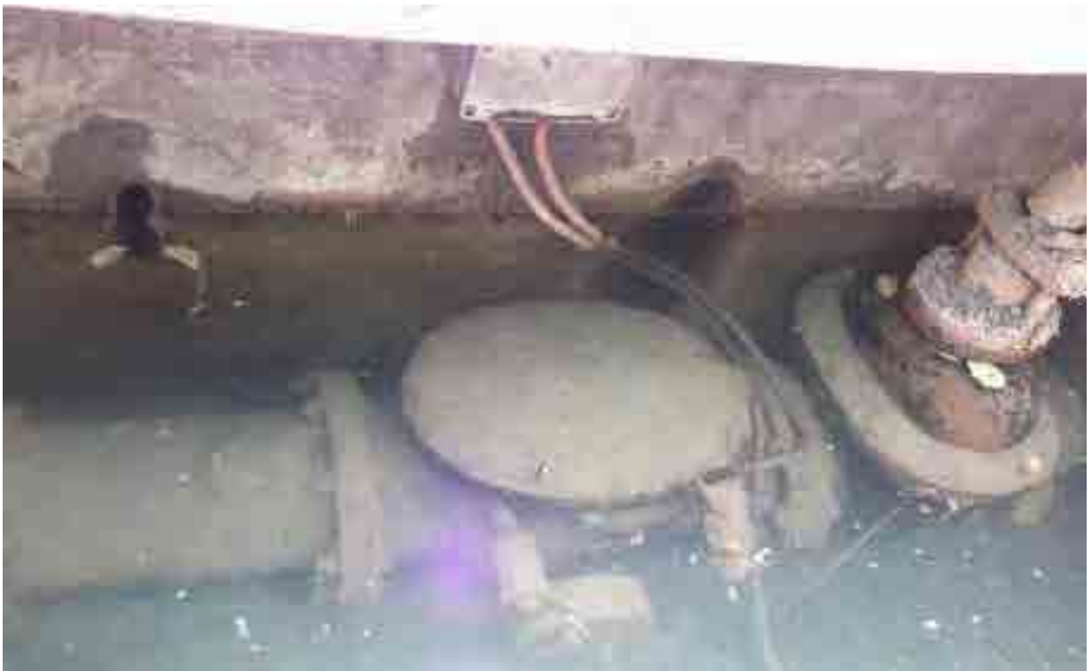
2b. Corrosion condition; medium level of corrosion occurring on steel
