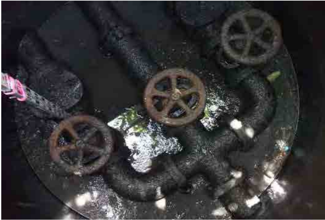
2b. Corrosion condition; there is corrosion in the valve pit steel pressure pipes 3.0 Manhole in front of one
