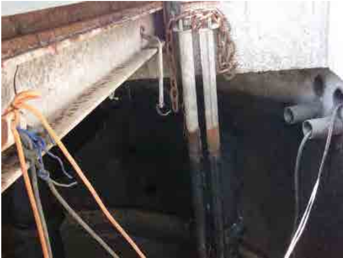
1c. Steel Rod Exposed; Corrosion not severe but starting
