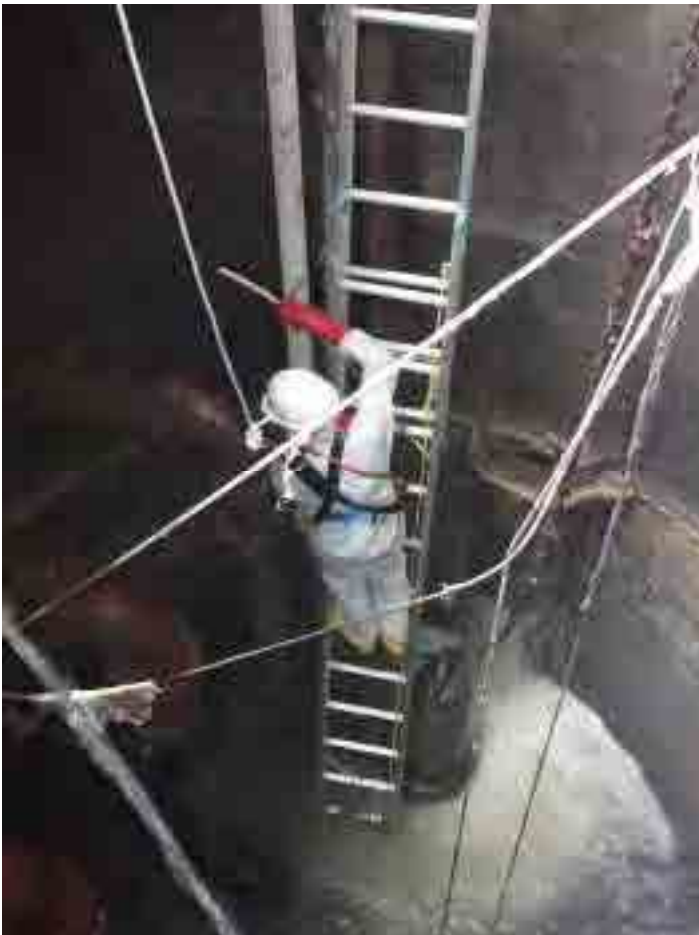
1b. Pump Pit Leakage Check; Not many leakages
