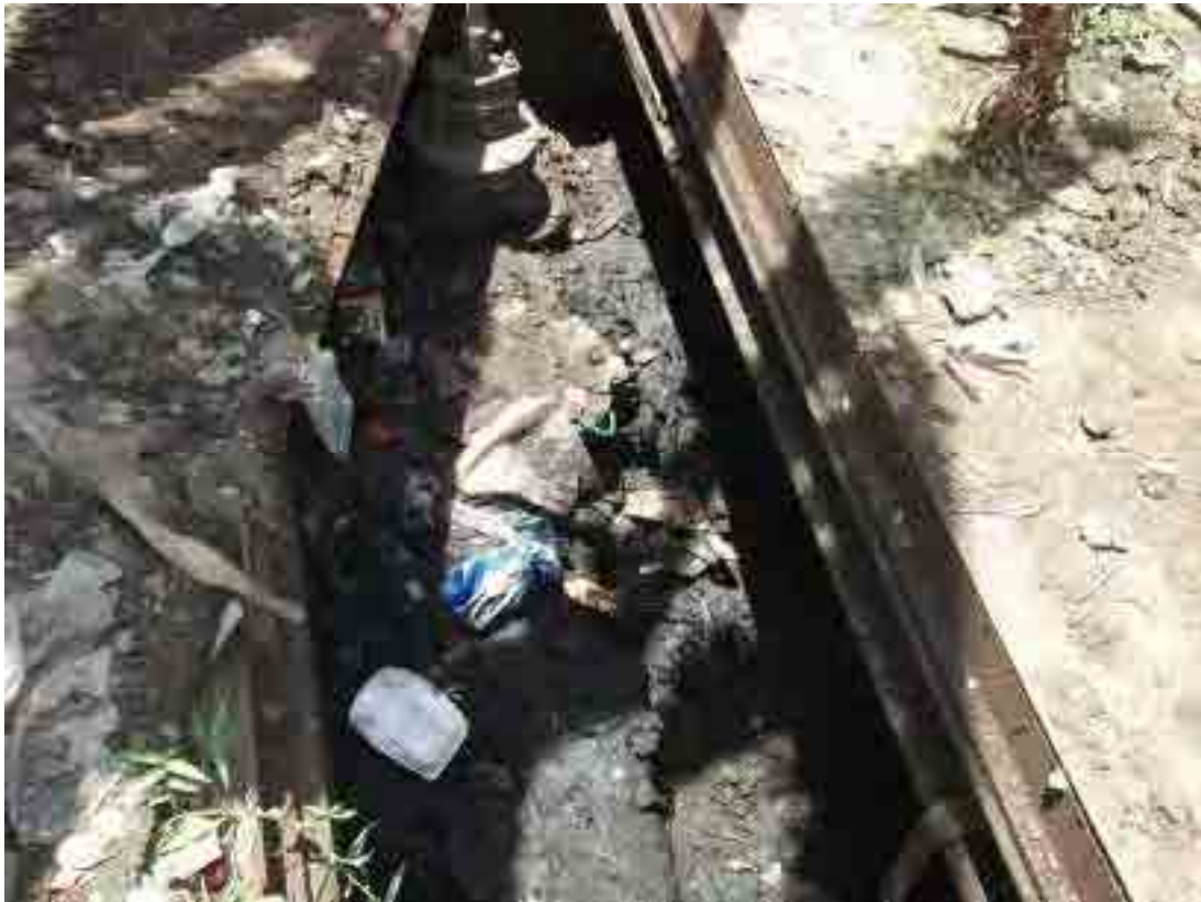
2b. Valve Pit covered with debris and rubbish
