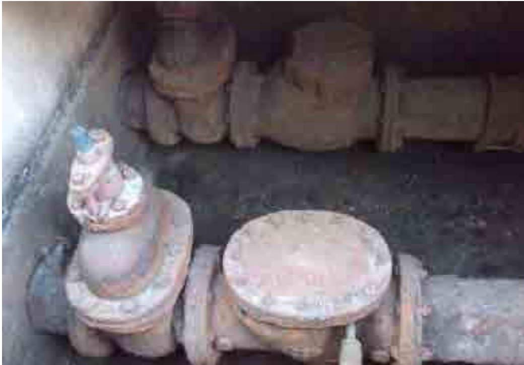
2b. Corrosion condition; Steel Pipes severely corroded.
