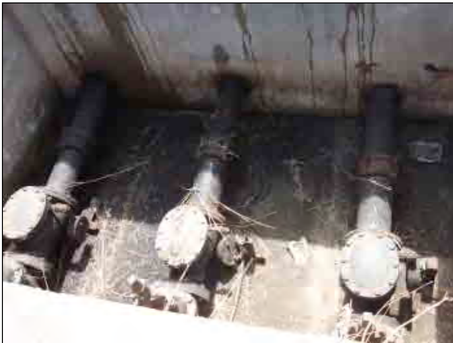
2a. Leakage condition; No major leakage at all
