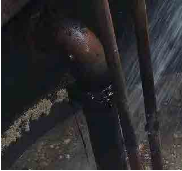
1c. Corrosion Condition; medium level of corrosion occurring on steel pipes
