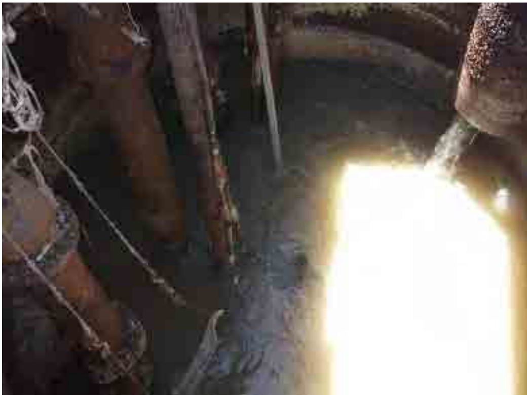
1d. Corrosion Check; All Steel Pipes badly corroded.
