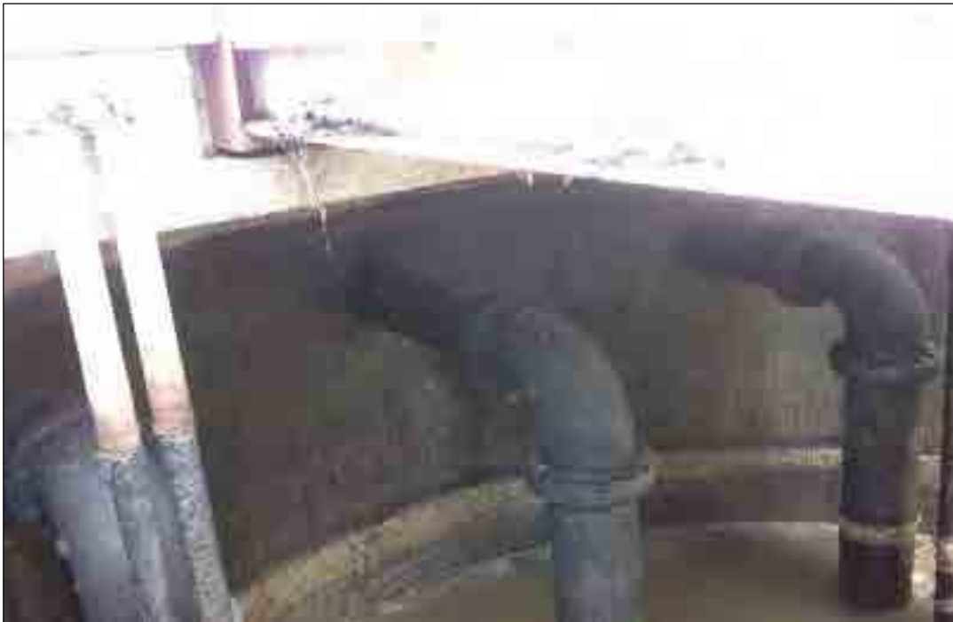
1b: Pump Pit Leakage Check; Not many leakages.
