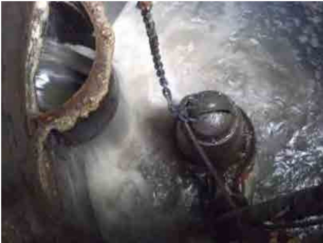
1d. Severe Place of Corrosion; Inflow pipe and pressure pipes
