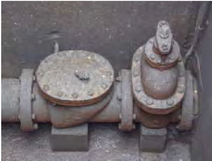
2c. Most steel pipes are severely corroded like this one.
