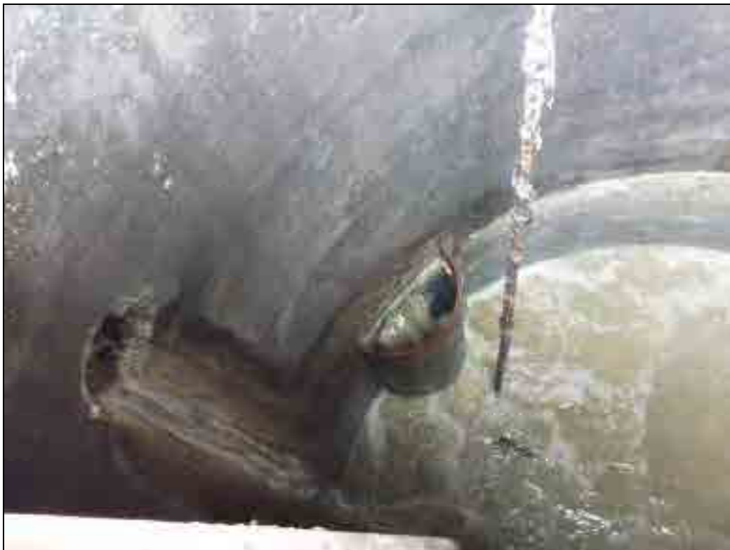
3a. Inflow Pipe 1 Top, PVC; Inflow Pipe 2 Bottom, Steel
