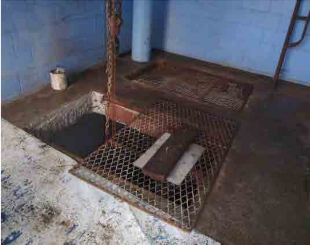
1g. Pump pit Slab Opening, Background is the Ventilation Pipe (Dia.
