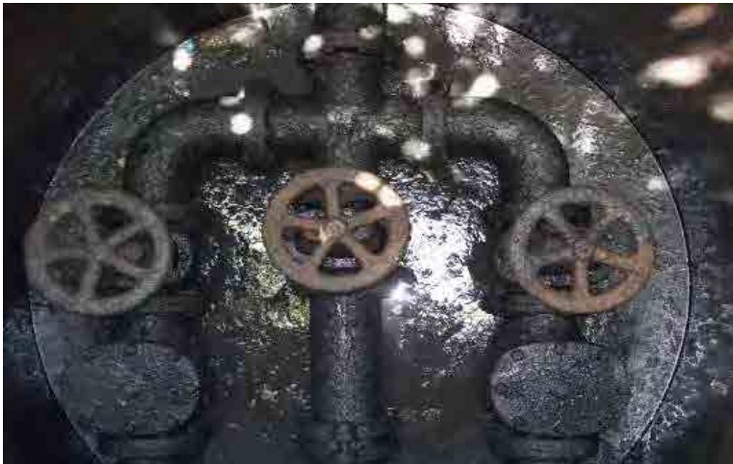
2a. Leakage condition; there is leakage in the valve pit
