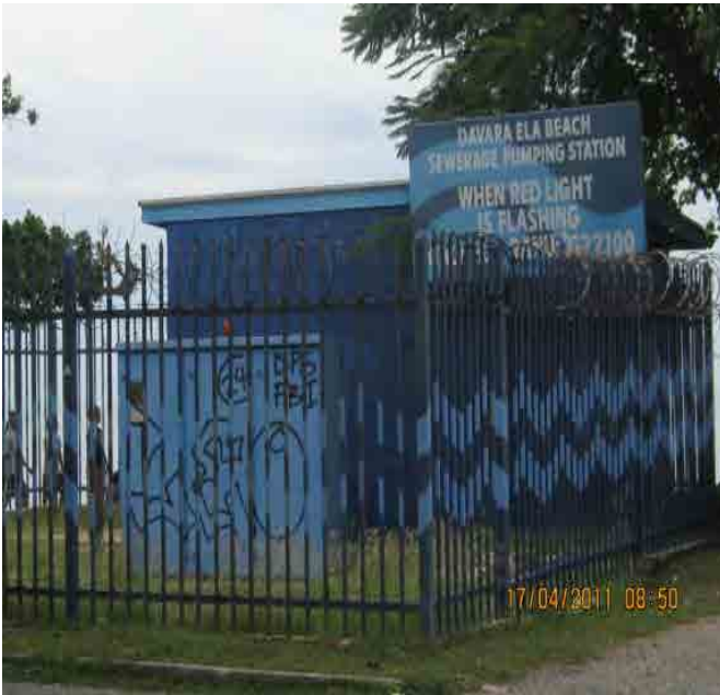
Existing pumping station
