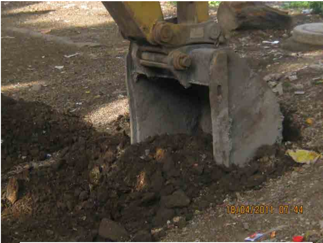
Excavation at PS Number 4
