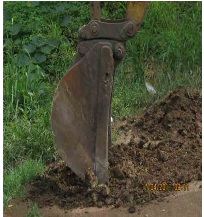
Excavation done using a backhoe
