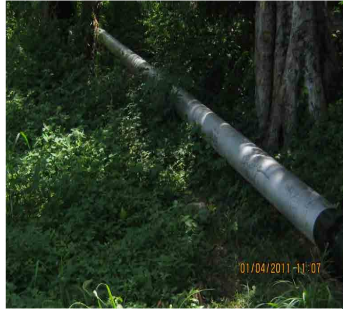
Inter Oil pipeline lying 3metres away from the proposed location
