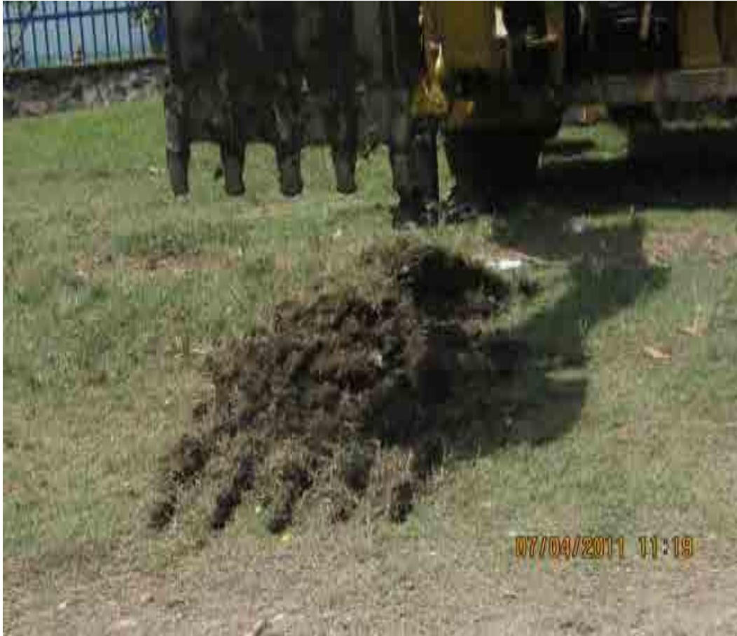
Excavation at PS No: 9
