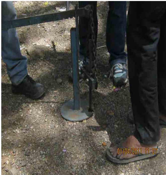
DCP Test done on Site
