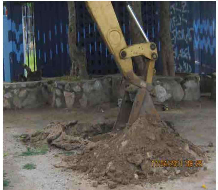
Excavation at the car park
