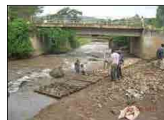
Construction of bank protection works
