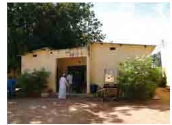
Existing Health Center (new center under construction through grant aid)
