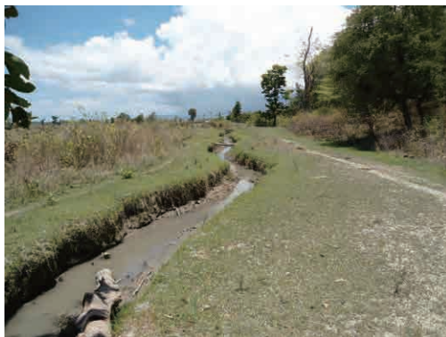
Existing irrigation canal (Canal is well maintained by farmers)
