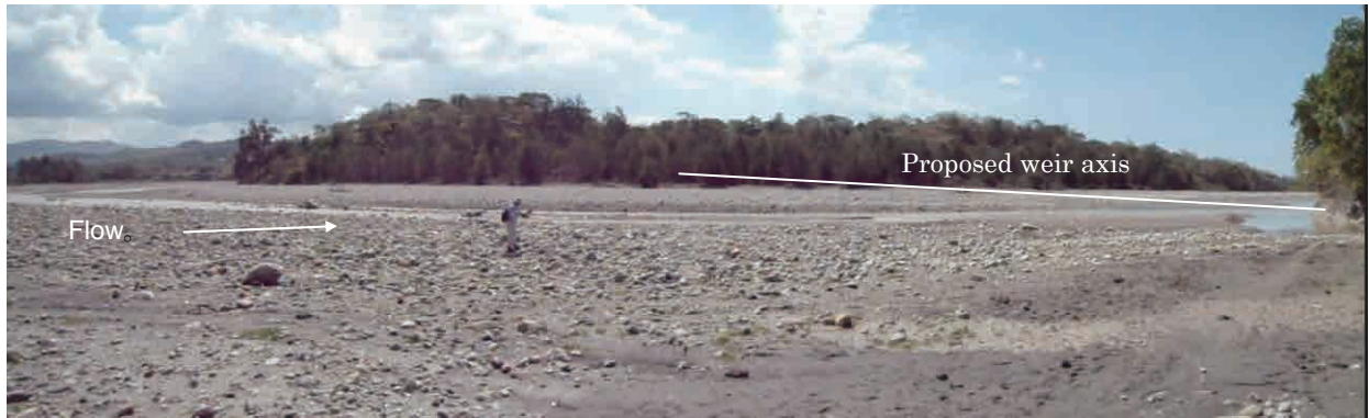
Proposed site of intake (Intake is installed at the most right side of the photograph)
