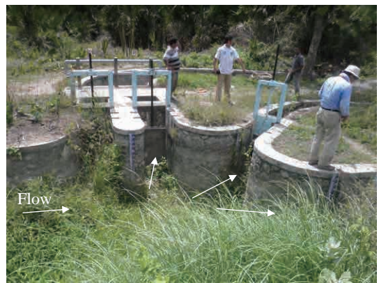
Diversion point (Diversion from main canal to secondary canals)
