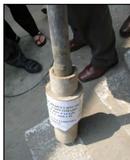
Photograph-3: Reduction with lead from asbestos cement to PVC in Comas. No suitable accessory.
