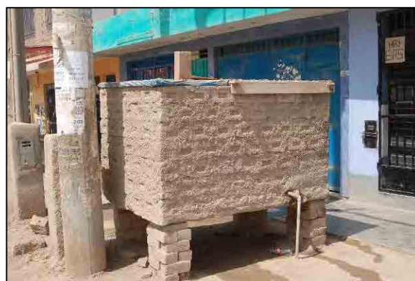
Picture 2.5.6-9: Typical Installation of Water Tank in Front of Home
