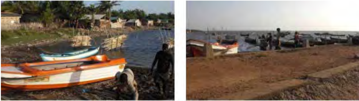
Figure 2.17: Navanturai Jetty: Before Rehabilitation
