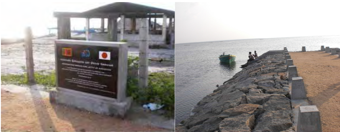
Figure 2.19: Kakkaitivu Jetty: After Rehabilitation
