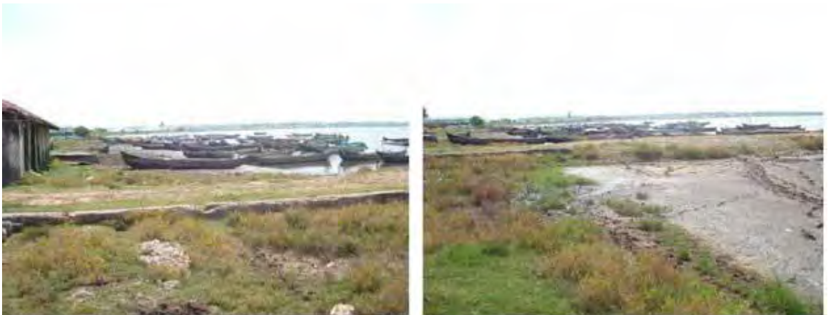
Figure 2.18: Kakkaitivu Jetty: Before Rehabilitation
