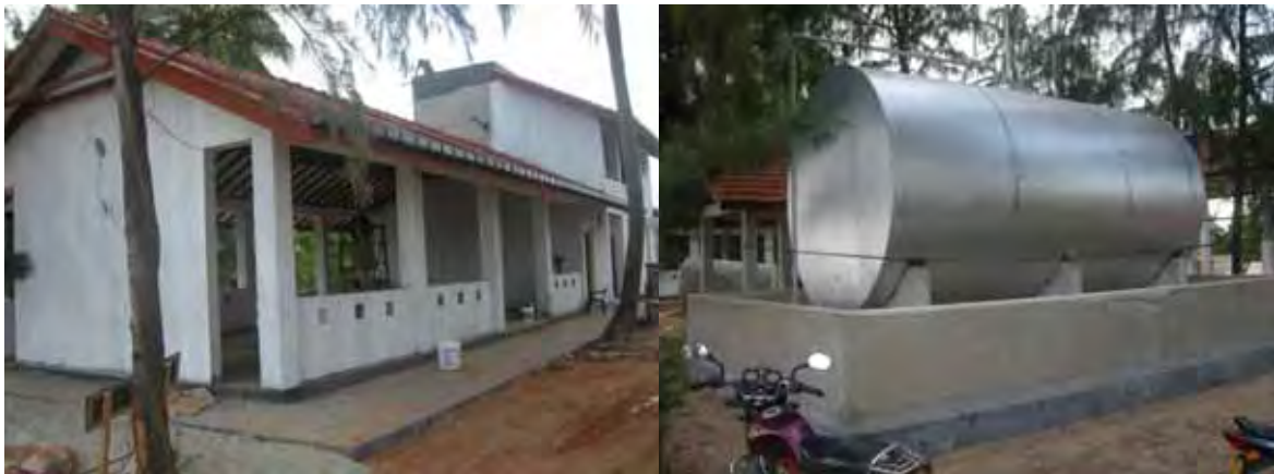
Figure 2.22: Shore Facilities constructed under IFAD/UNOPS Project in Kaluwankerni Landing Site, Batticaloa District
