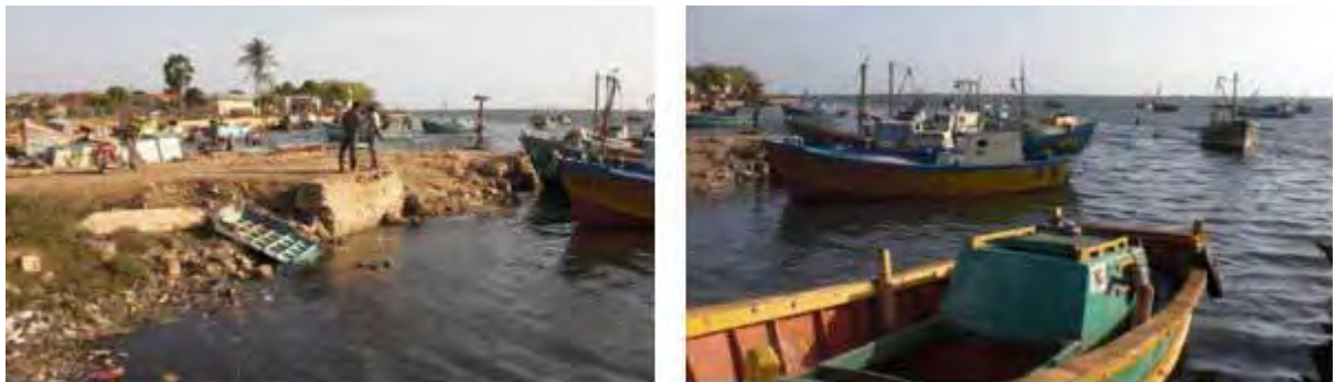
Figure 2.13: Gurunagar Landing Site
