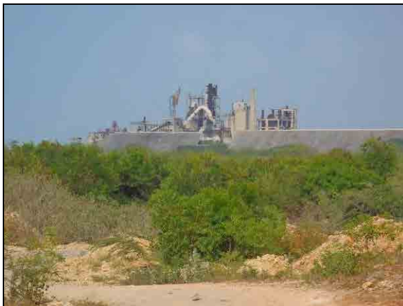
Inoperative Cement Factory in KKS
