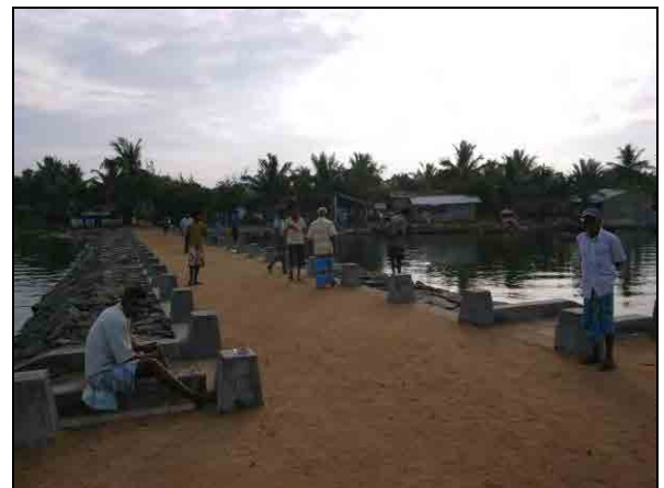
Jetty Renovation (After)
