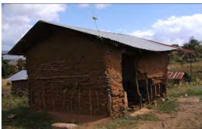
Figure Fig 3.3: Wooden frame, clay plastered wall, iron sheet roof structure in Hodi B
