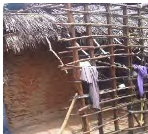
Figure 3.2: Wooden Frame, Clay Plastered Wall, Thatch Roof
