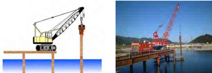
Figure 9.2-2 Concept of Temporary Bridge
