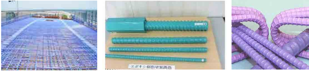
Figure 9.4-1 Epoxy Coated Reinforcing Bars
