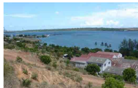
Figure 6.1-3 Mombasa New Container Terminal Construction Site
