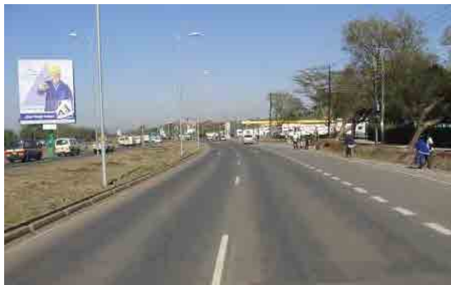
Figure 5.2-1 Section of the Completed Lanet - Njoro Turn Off / Dual Carriageway Road (A104)
