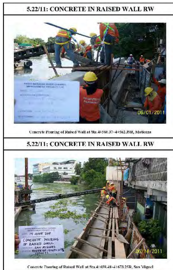
Figure 3.4 Revetment Works (Photo by Toyo, June 2011)
