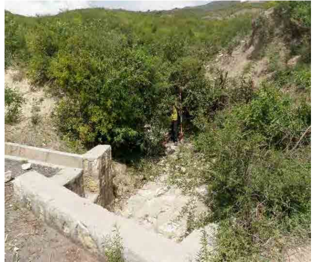
Photo 3. 9.45 Entire picture of MS016 (upstream from the road)
