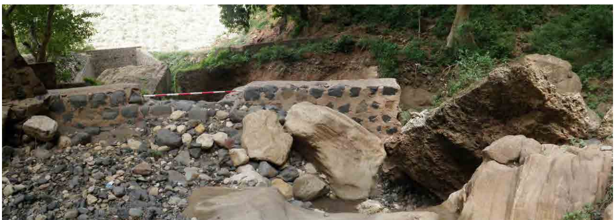
Photo 3. 9.72 Dam built upstream from the road (picture taken from the upstream)
