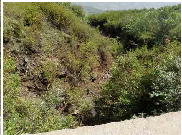
Photo 3. 9.5 Entire picture of MS002 (the downstream from the road)
