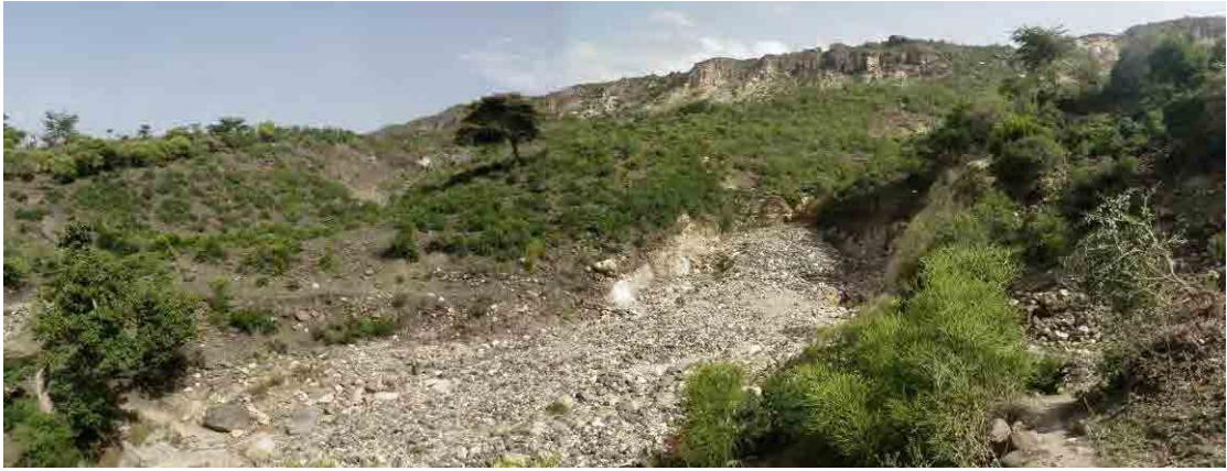
Photo 3. 9.14 Channel upstream (covered with rock blocks)
