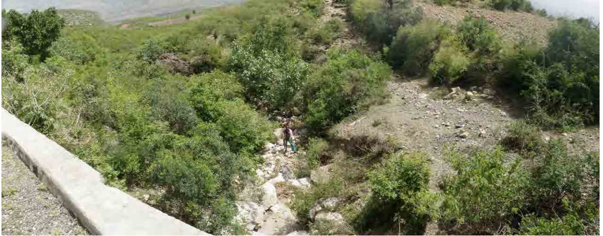
Photo 3. 9.29 Entire picture of MS010 (at downstream from the road)
