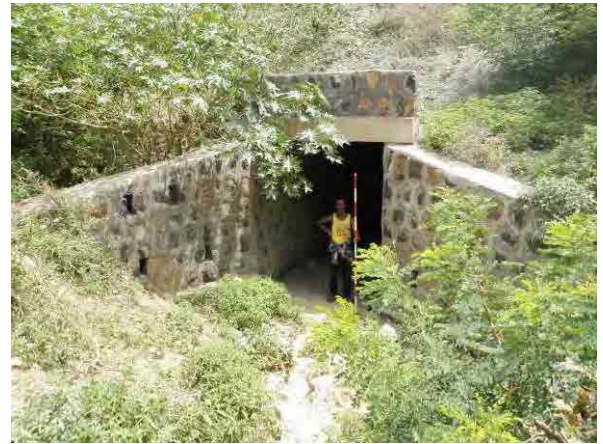
Photo 3. 9.35 Box culvert installed under the road
