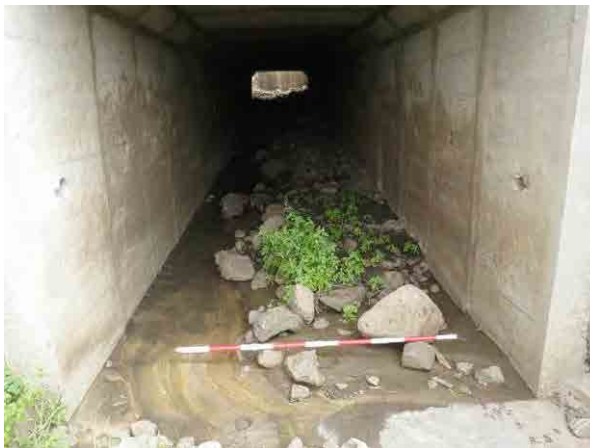
Photo 3. 9.94 Box culvert (upstream direction)
