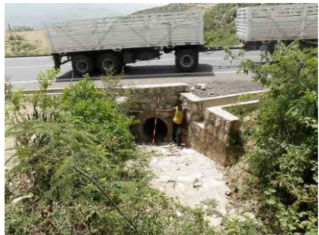
Photo 3. 9.47 Drainage pipe installed under the road
