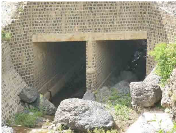
Photo 3. 9.108 Box culvert installed under the road
