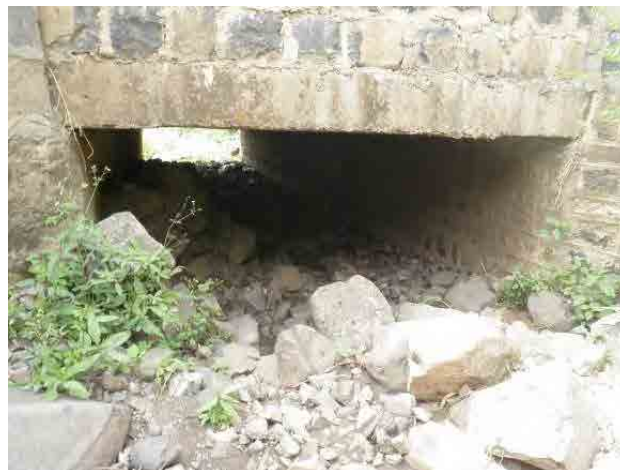
Photo 3. 9.98 Box culvert installed under the road (crushed rocks deposit)
