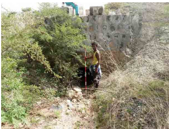
Photo 3. 9.63 Drainage pipe installed under the road
