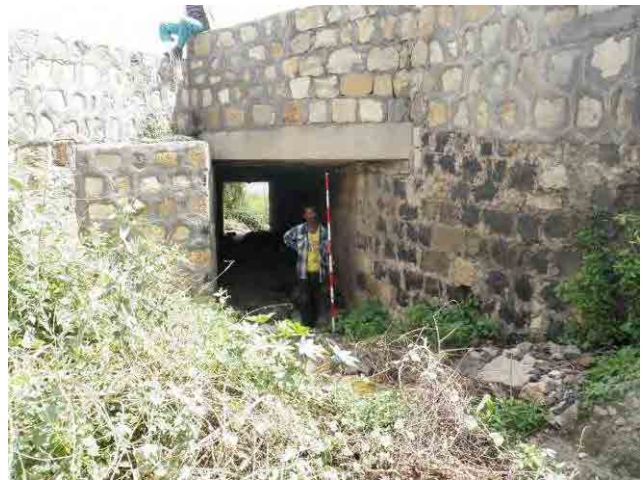
Photo 3. 9.27 Box culvert installed under the road (no sediment deposits)
