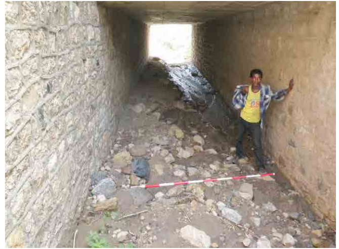
Photo 3. 9.24 Entire picture of MS009 (upstream from the road) Photo 3. 9.25 Box culvert installed under the road
