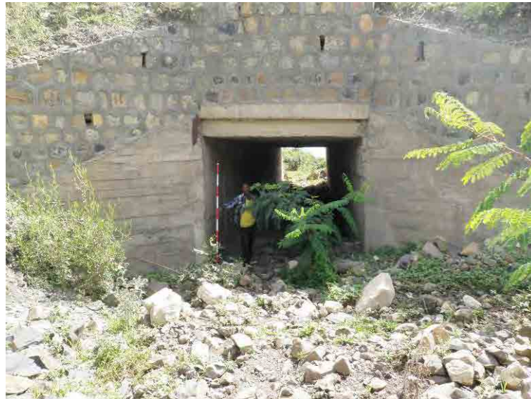
Photo 3. 9.23 Box culvert installed under the road (rock blocks are distributed)
