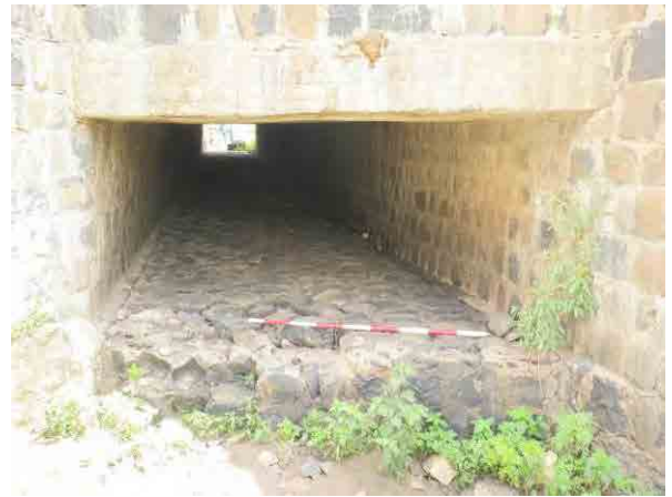
Photo 3. 9.114 Inside the box culvert
