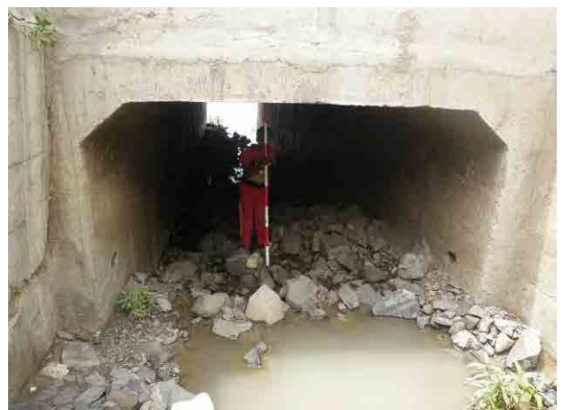
Photo 3. 9.101 Box culvert (crushed rocks deposit)
