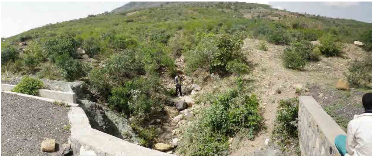
Photo 3. 9.28 Entire picture of MS010 (upstream from the road; no water flow)
