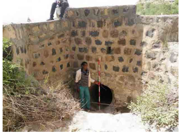
Photo 3. 9.54 Drainage pipe installed under the road
