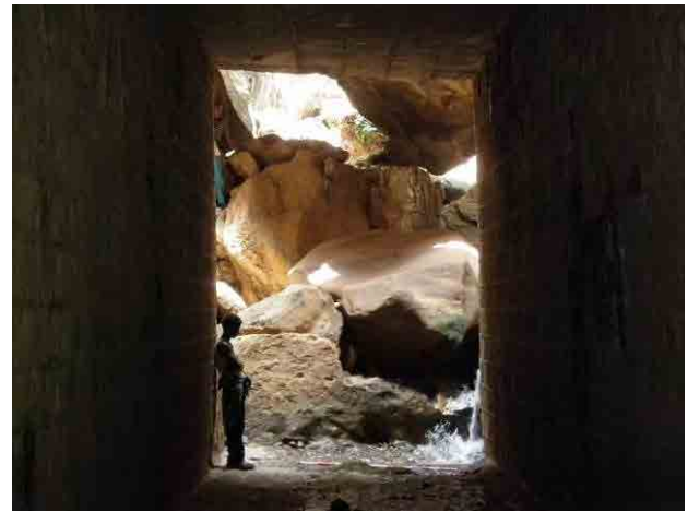
Photo 3. 9.74 Inside view of the box culvert
