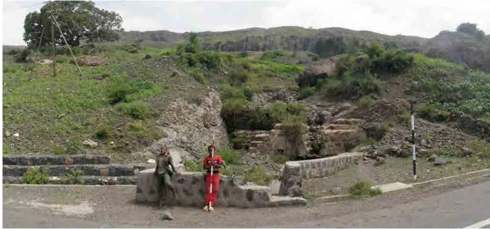
Photo 3. 9.99 Entire picture of MS031 (upstream from the road)
