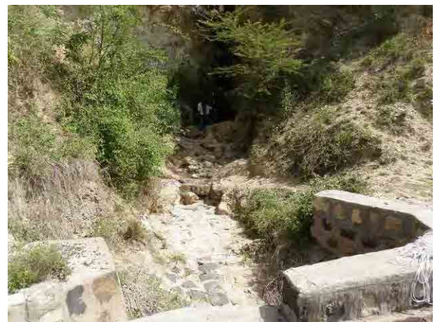
Photo 3. 9.52 Entire picture of MS018 (upstream from the road)
