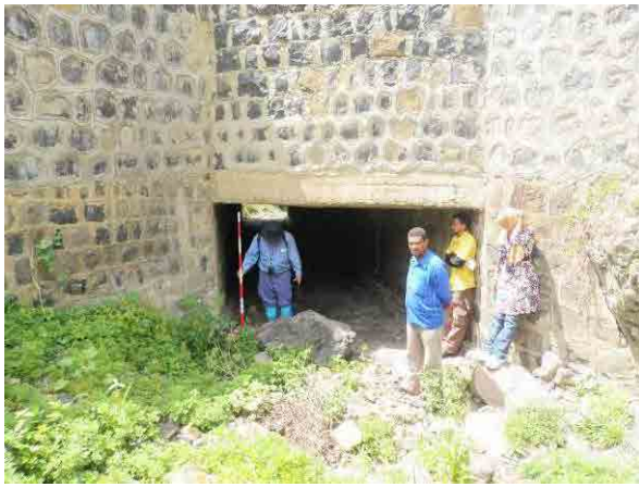
Photo 3. 9.113 Box culvert installed under the road
