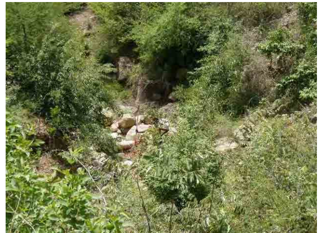
Photo 3. 9.42 Entire picture of MS015 (upstream from the road)
