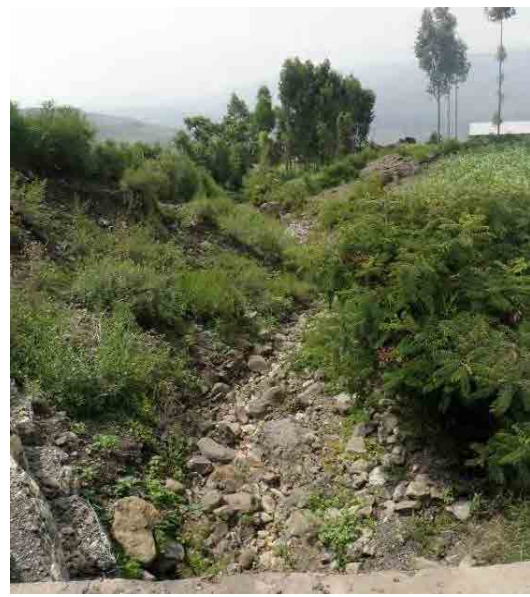
Photo 3. 9.97 Entire picture of MS030 (at downstream from the road)
