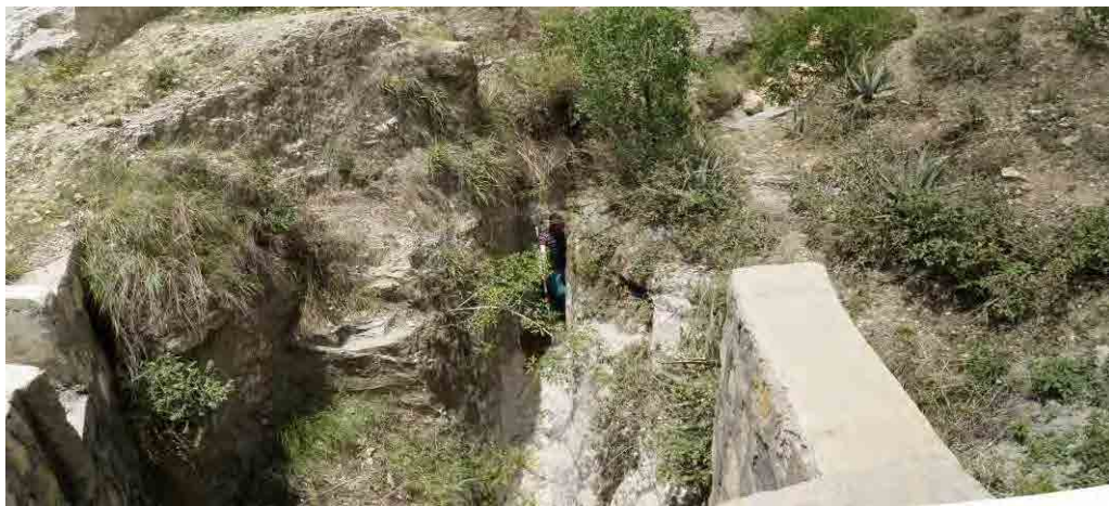
Photo 3. 9.36 Entire picture of MS013 (upstream from the road; no water flow)
