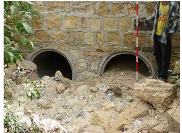
Photo 3. 9.60 Drainage pipes installed under the road
