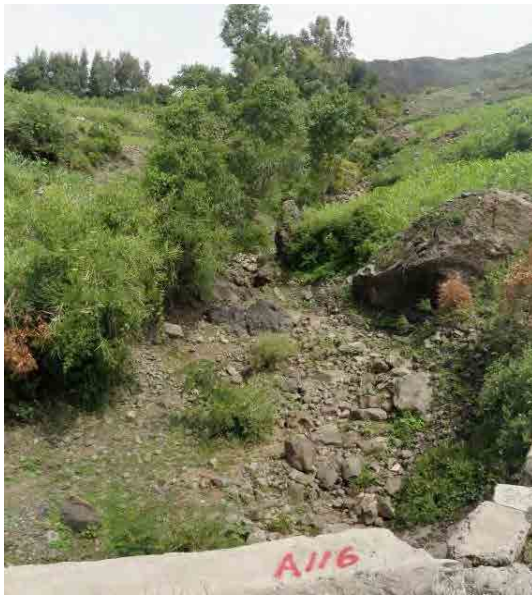
Photo 3. 9.96 Entire picture of MS030 (upstream from the road)
