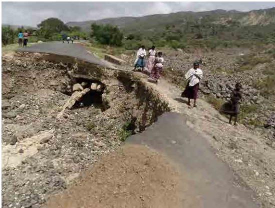
Photo 3. 9.15 Damaged bridge
