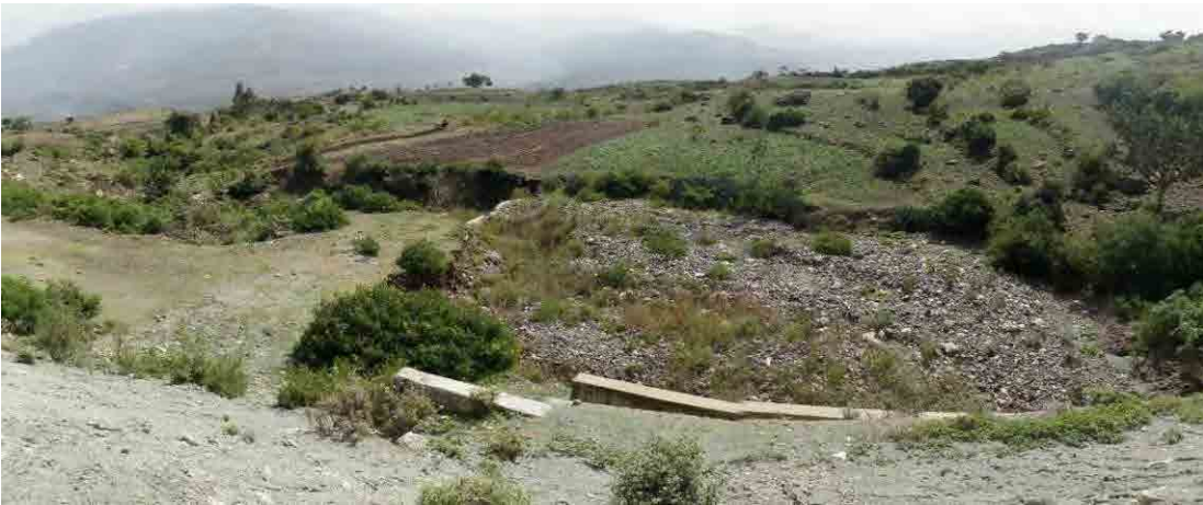
Photo 3. 9.20 Entire picture of MS007 (downstream from the road; behind the dam is almost filled with sand)
