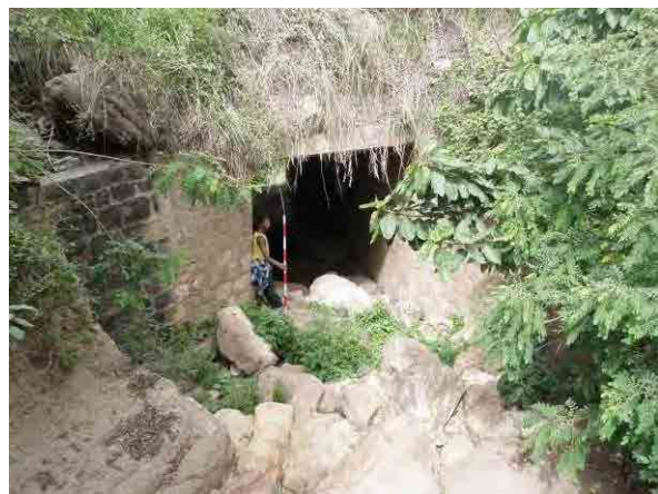
Photo 3. 9.67 Box culvert installed under the road
