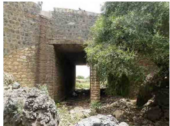
Photo 3. 9.16 Box culvert (with rock blocks deposited)
