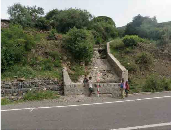
Photo 3. 9.91 Entire picture of MS029 (upstream from the road)
