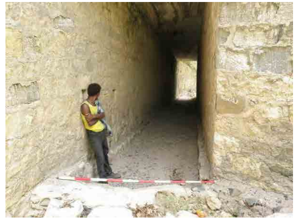
Photo 3. 9.44 Box culvert installed under the road
