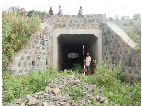
Photo 3. 9.95 Box culvert (downstream direction)
