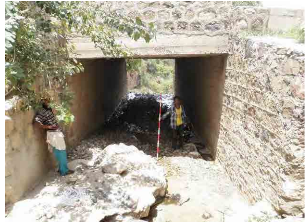
Photo 3. 9.84 Box culvert under the road
