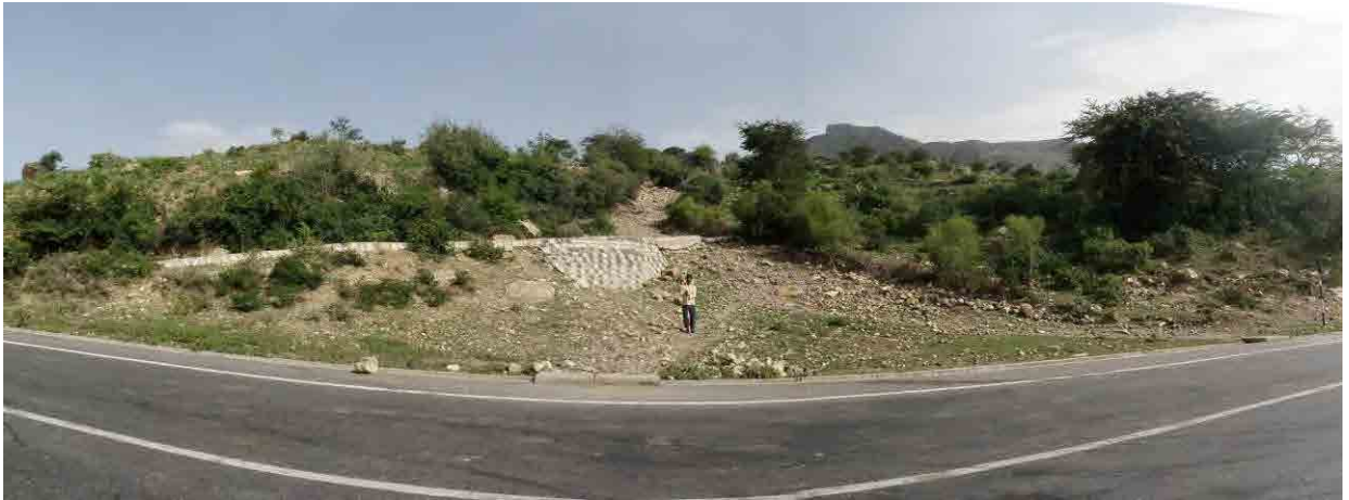
Photo 3. 9.17 Entire picture of MS006 (upstream from the road; water flow is drained from trenches to gutters on the road side)
