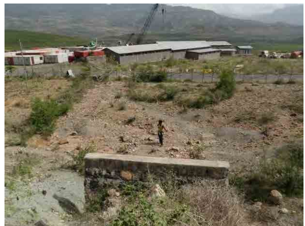
Photo 3. 9.64 Entire picture of MS021 (downstream from the road)
