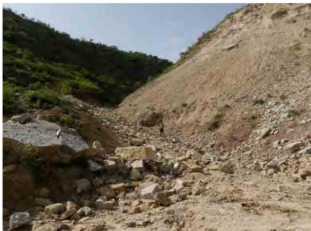
Photo 3. 9.59 Quarry on the left bank
