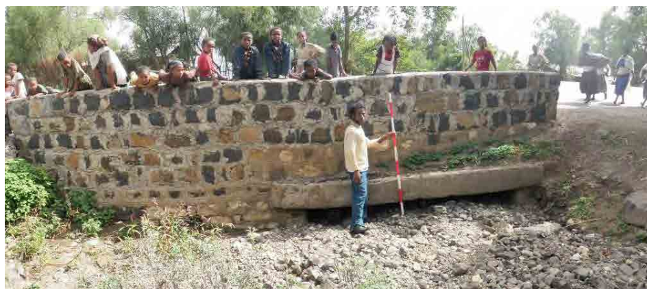
Photo 3. 9.10 Box culvert installed under the road (blocked by rock blocks)
