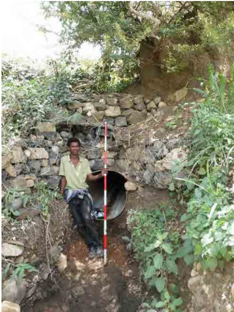
Photo 3. 9.85 Drainage pipe installed in the channel upstream
