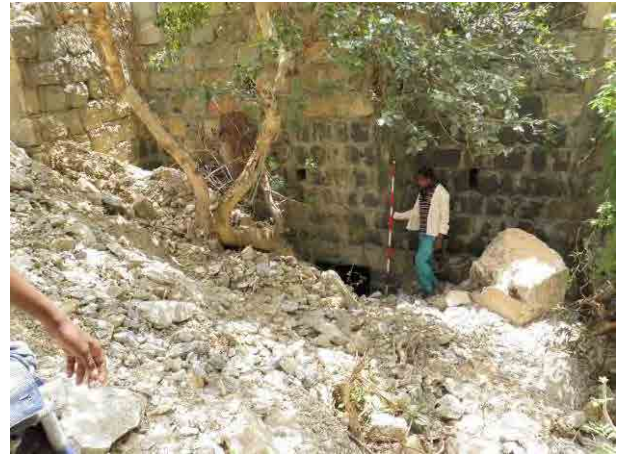
Photo 3. 9.41 Box culvert installed under the road
