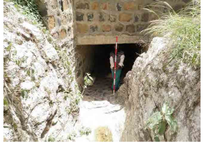
Photo 3. 9.38 Box culvert installed under the road
