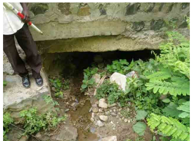
Photo 3. 9.90 Box culvert installed under the road
