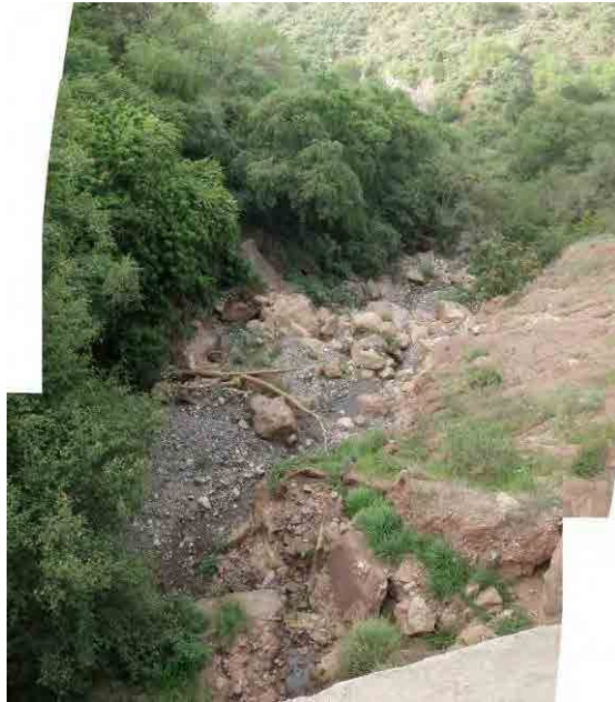
Photo 3. 9.73 Entire picture of MS023 (downstream from the road)
