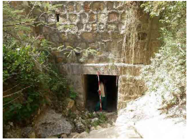
Photo 3. 9.57 Box culvert installed under the road
