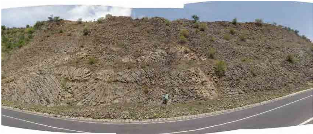
Photo 3. 8.8 Conditions of joints and cracks developing on the cut slope
