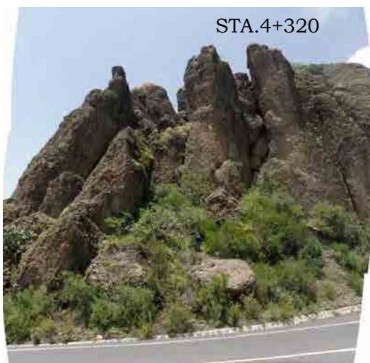
Photo 3. 8.9 Unstable basaltic outcroppings
