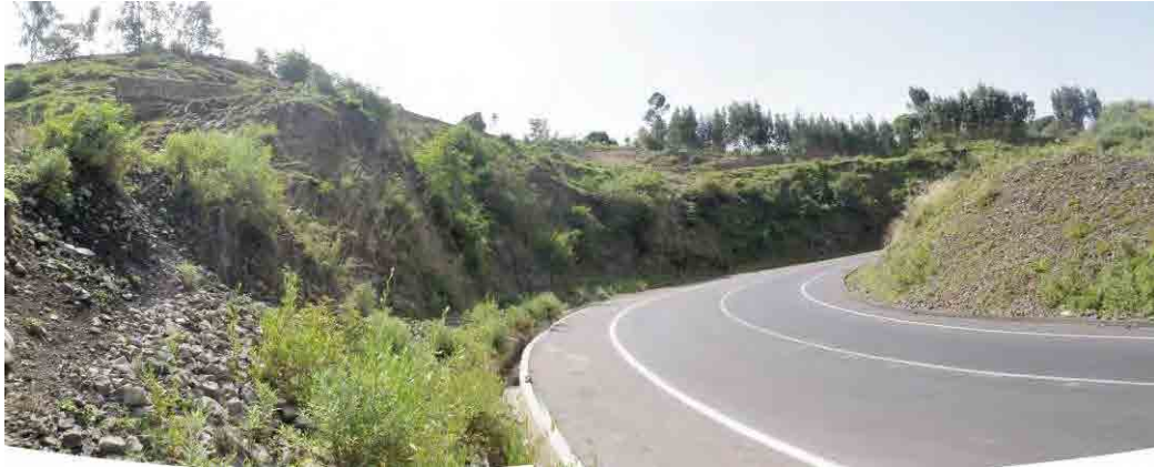
Photo 3. 8.38 Weathered basaltic cut slopes
