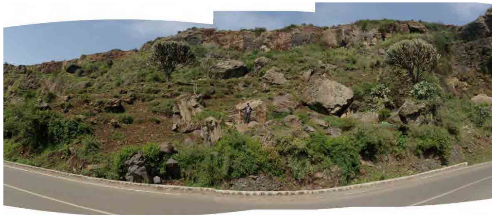
Photo 3. 8.5 Fallen rocks distributed at the bottom (1m – 3m in diameter)
