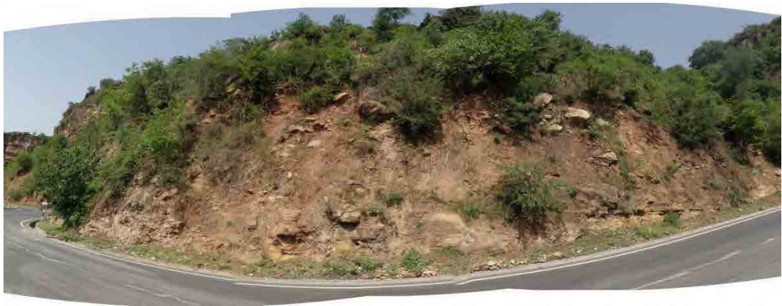
Photo 3. 8.28 Detached rocks distributing on cut slopes
