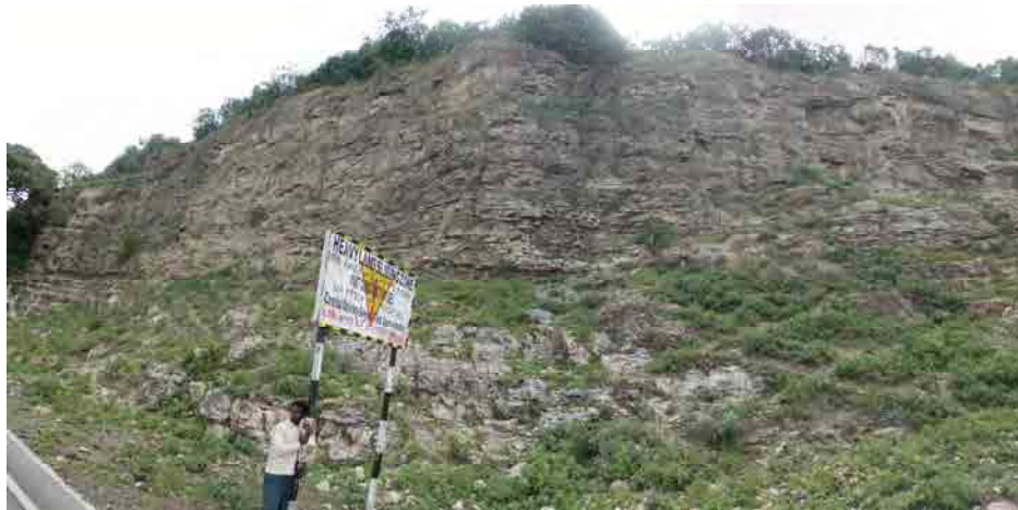
Photo 3. 8.31 Fallen rocks distributed on the bottom of the cliffs
