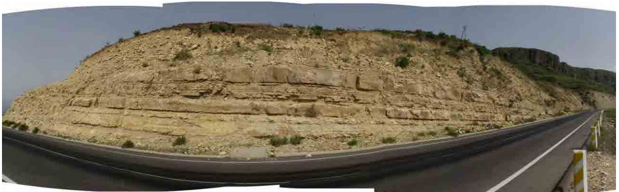
Photo 3. 8.35 Weathered limestone cut slope
