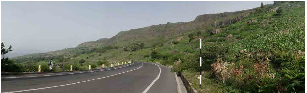
Photo 3. 8.32 Entire picture of section RF0013 (taken from the section end point)
