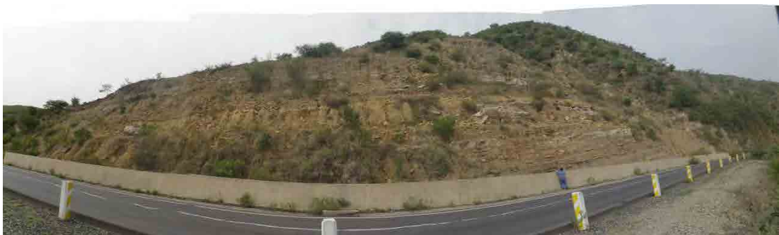
Photo 3. 8.17 Retaining wall on the section start side (1.5m high, extending 100m)
