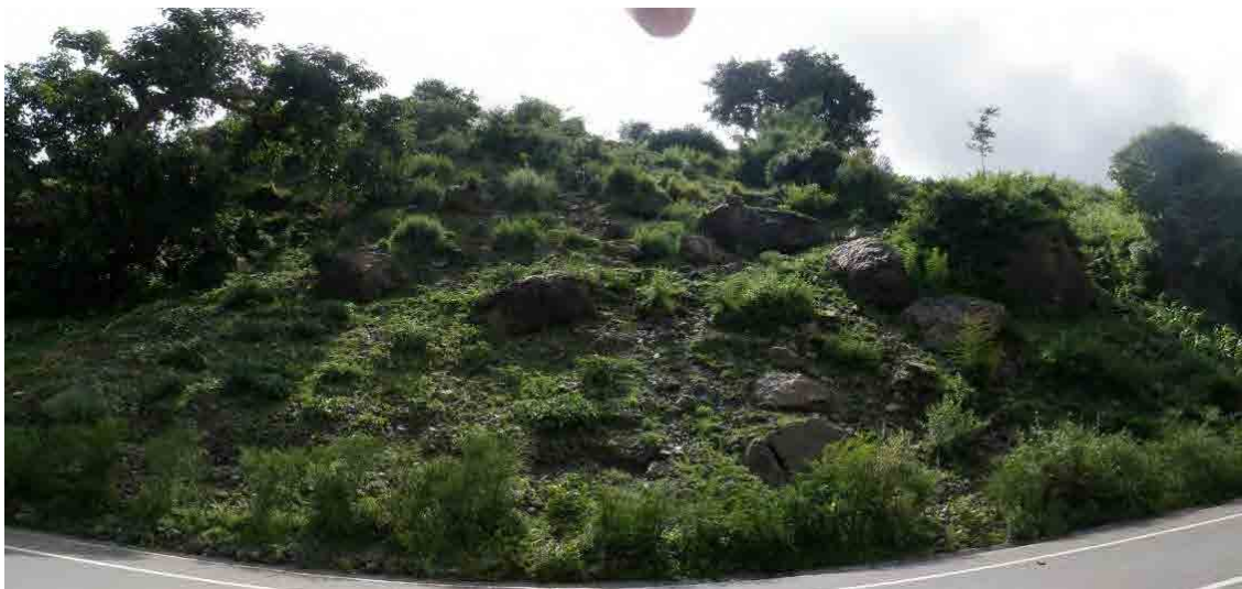
Photo 3. 8.33 Detached rocks distributed on the slopes
