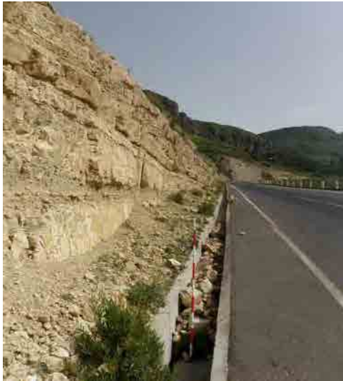
Photo 3. 8.34 fallen rocks distributed at the bottom of the cut slope
