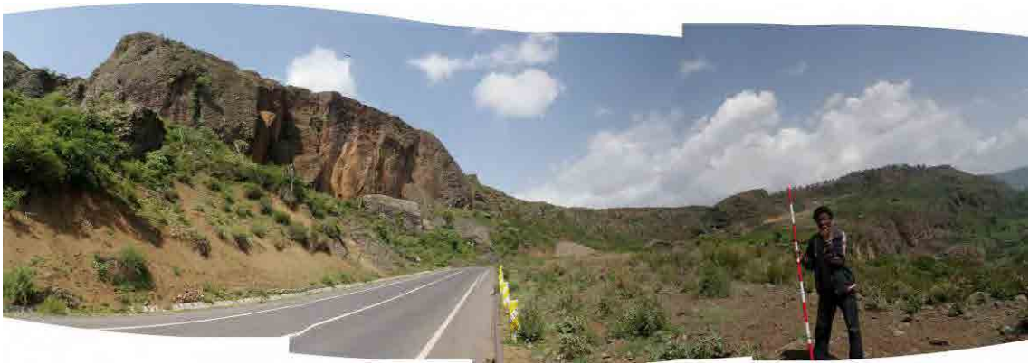
Photo 3. 8.6 Entire picture of section RF003 (taken from the section end)
