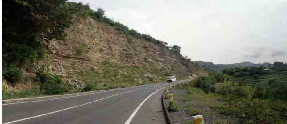
Photo 3. 8.30 Entire picture of section RF0013 (taken from the section start point)
