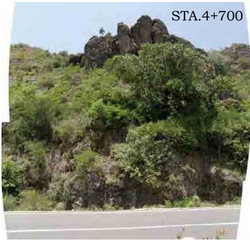
Photo 3. 8.11 Unstable basaltic outcroppings
