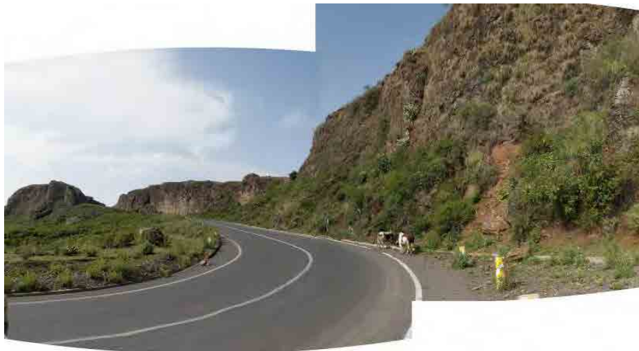
Photo 3. 8.2 Entire picture of section RF001 (taken from the section end point)
