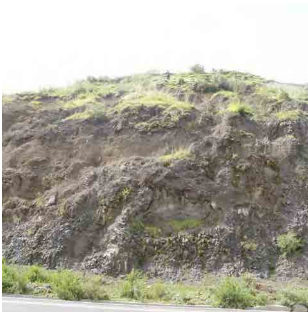
Photo 3. 8.36 Weathered basaltic cut slope
