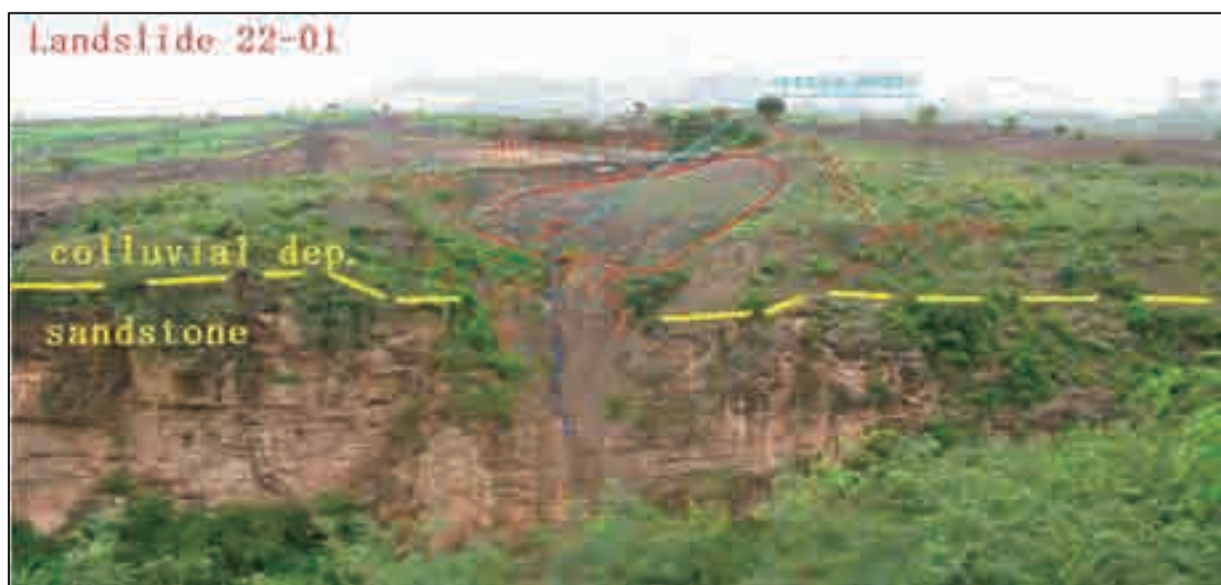
Photo 4.4.32 Landslide 22-01 from opposite side terrace cliff.
