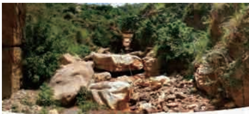
Photo 6.3.16 On-site survey of stream bed
