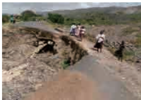
Photo 4.8.2 Overflowed sediment at S09-1
