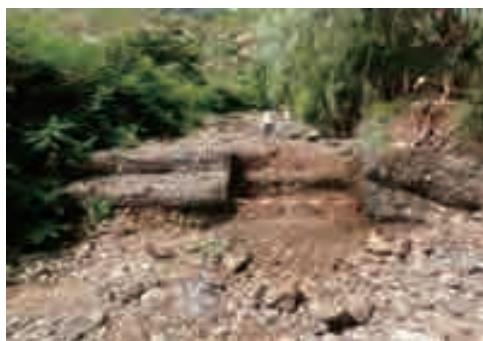
Photo 4.8.1 Overflowed sediment at S08-2
