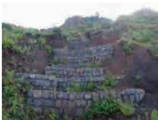
Photo 5.4.5 Gabions installed in streambed
