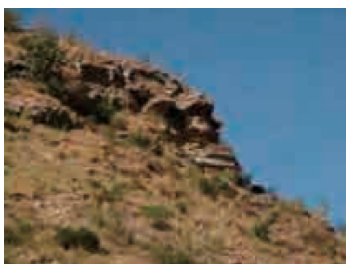
Photo 5.4.9 Rockfall from a Natural Slope
