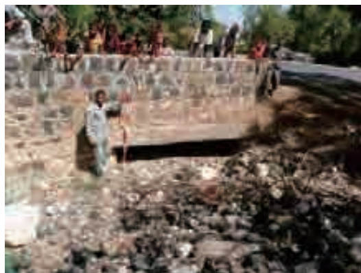
Photo 5.4.11 Insufficient Drainage Processing Photo 5.4.12 Blocking of a Box Culvert
