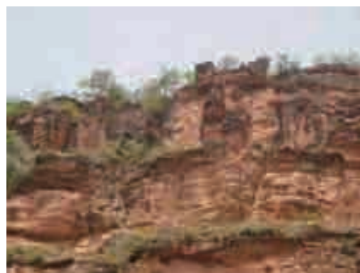
Photo 5.4.8 Detached-away Type Rockfall
