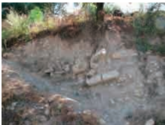
Photo 4.4.26 The colluvial deposit mixed up with sliding soil
