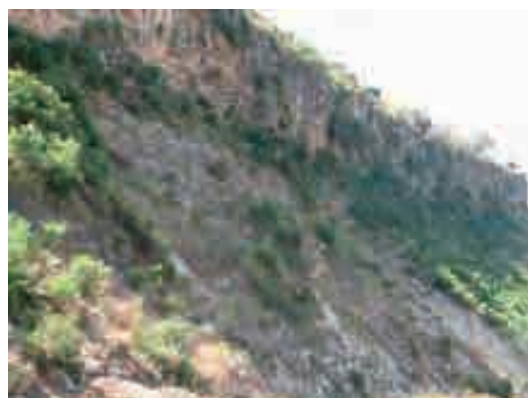
Photo 4.4.20 The lower limestone forms gentle slope
