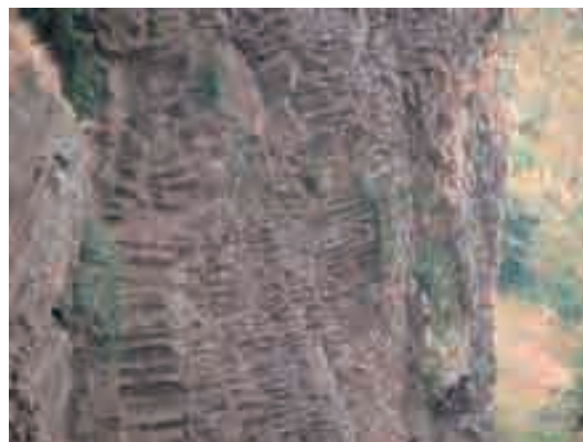
Photo 4.4.11 Clearly developed columnar joints which are mainly horizontal direction
