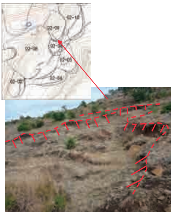
Figure 4.3.19 New Cracks at the Head of L/S02-09
