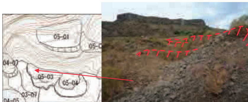
Figure 4.3.21 Landslide Area at L/S05-03
