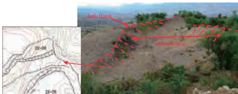
Figure 4.3.28 L/S28-05 Left Flank Where Landslide is Clearly Shown at L/S28-05
