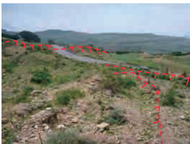
Photo 4.3.1 Depression Zone at Upper part of Landslide
