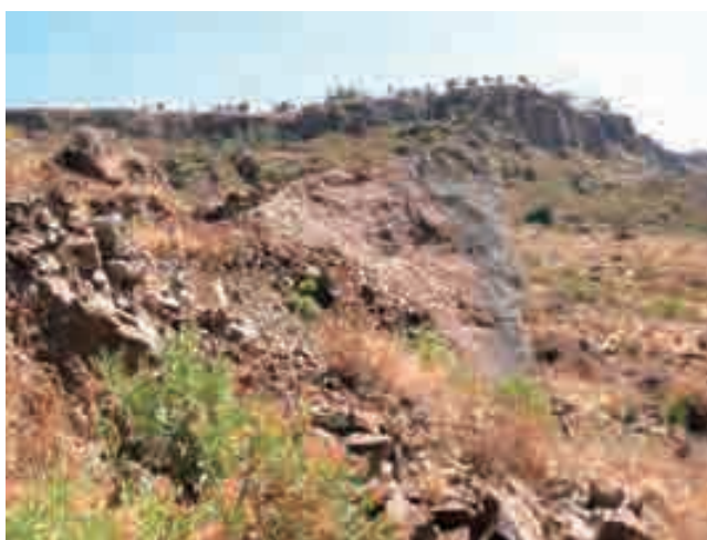
Photo 4.3.4 Ridge Caused by Compression Force of Landslide
