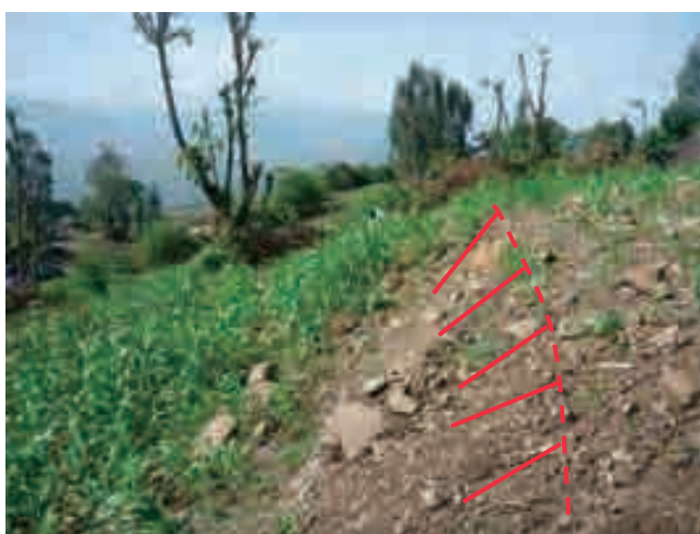
Photo 4.3.3 Step Caused by Landslide
