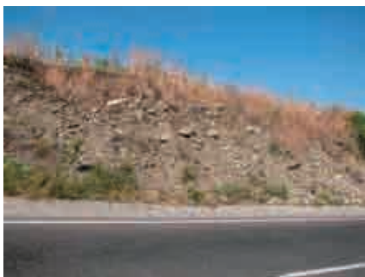
Photo 4.4.24 Colluvial deposit composed of gravel, sand, mud and clay
