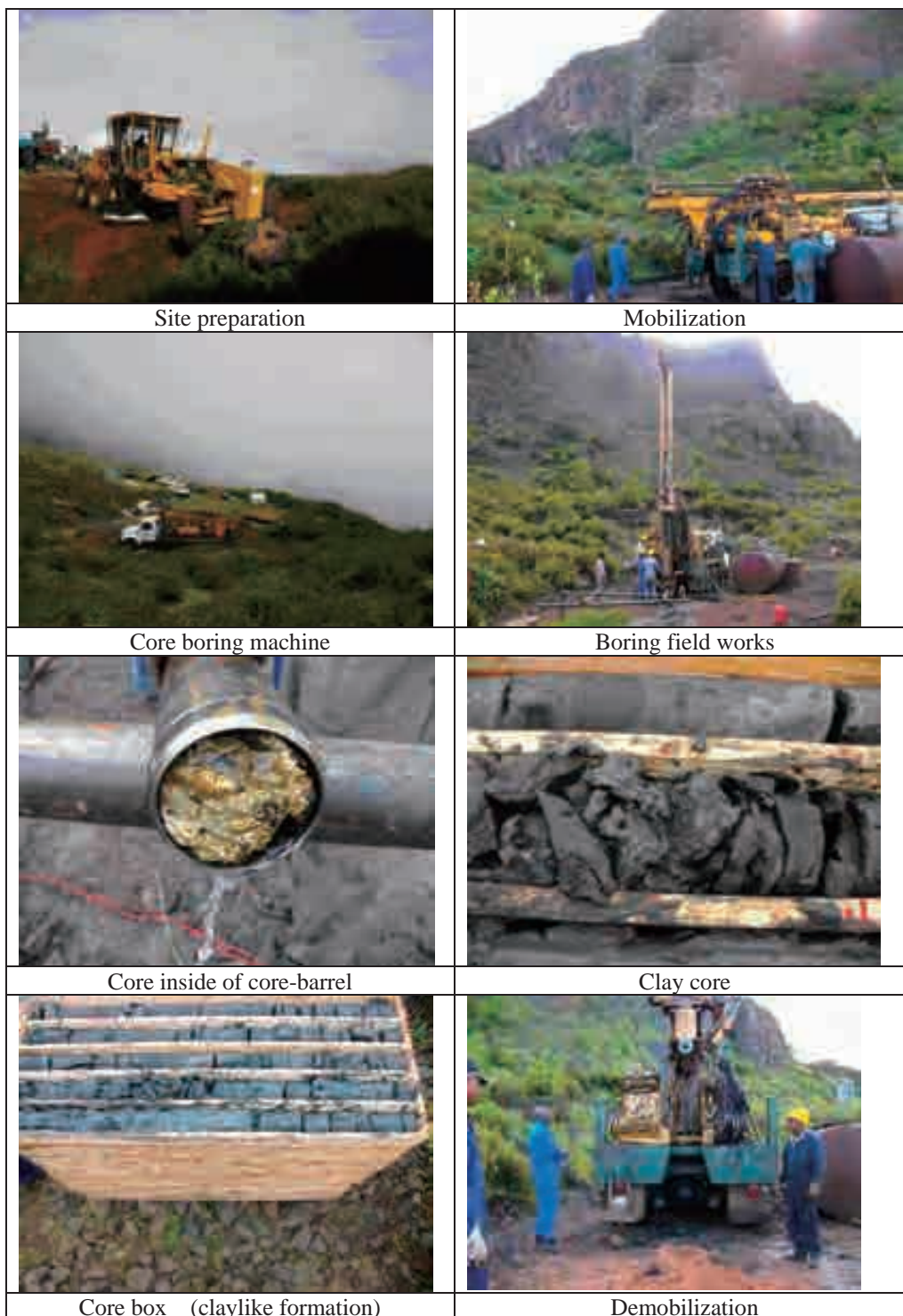
Photo 3.7.1 Field photograph for the core boring procedures
