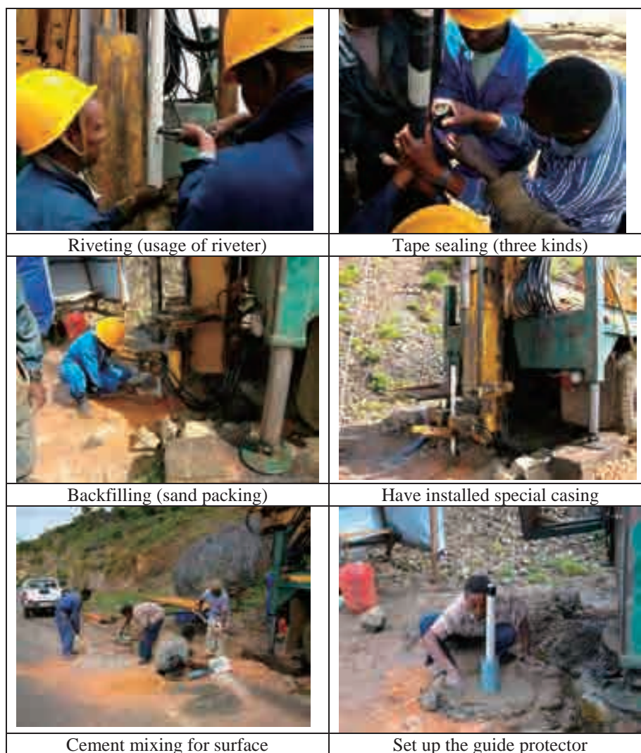
Photo 3.7.4 Field photograph for the inclinometer (2)
