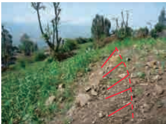
Photo (1) Displacement on the L/S208-1
