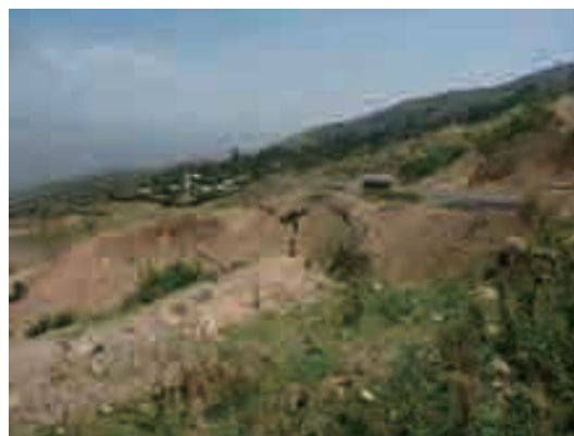
Photo 2.1.8 Gentle slope between 1,700 and 1,980 m with many landslides apparent
