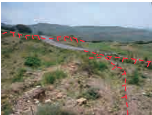
Photo (1) Main scarps and subsidence in the L/S28-3 (1). A new and clear main scarp with about 10 m difference is continuing, and the displacement is also occurring on the road. On the valley side, cracks, whose mountain side is sinking, that runs roughly in parallel with the main scarps.
