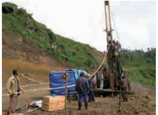
Drilling work at ST.0.800
