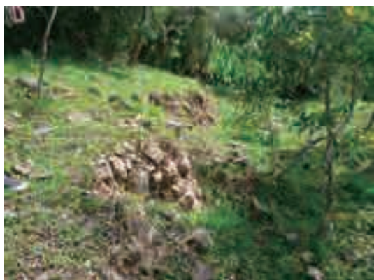
Photo (3) Crack at the head of the L/S28-1 (2).
