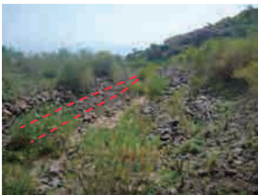
Photo (3) A continuous crack along the channel in the L/S05-1 The crack continues along the old channel.
