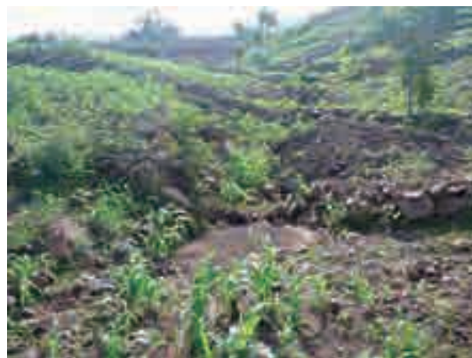
Photo (8) Channel on the L/S27-2. There is a series of small channel.
