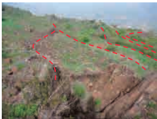
Photo (3) Cracks near the boundary of the toe of L/S00-1 and L/S00-3. The maximum difference in level of the cracks is about 2m. The transported land mass could also be seen to have taken on a toppling style.
