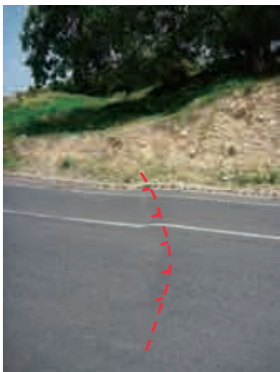
Photo (1) Main scarps and subsidence in the L/S28-3 (1). A new and clear main scarp with about 10 m difference is continuing, and the displacement is also occurring on the road. On the valley side, cracks, whose mountain side is sinking, that runs roughly in parallel with the main scarps.
