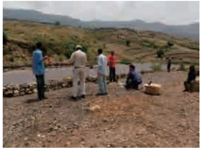
Installation of groundwater level meter, 22 nd Jun. 2011
