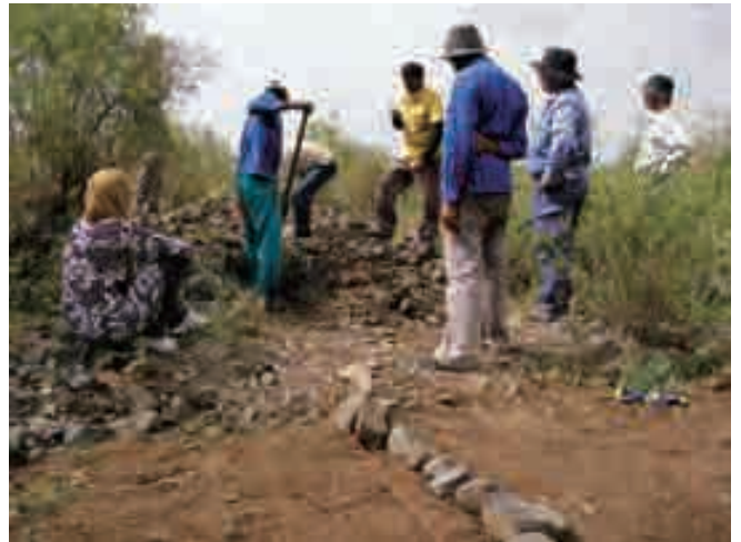
Digging trench for extensometer
