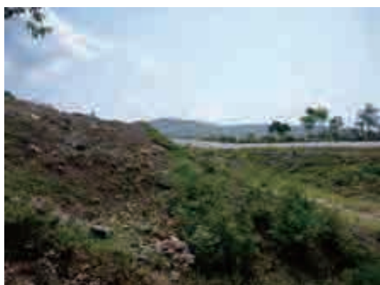
Photo (5) Subsidence on the head of the L/S28-1.
