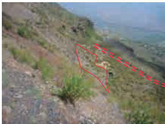
Photo (1) L/S05-1 block as viewed from the top An old channel crosses the L/S05-1, and debris from the upper part is piled up on the block. The debris is a load on the L/S05-1 block.
