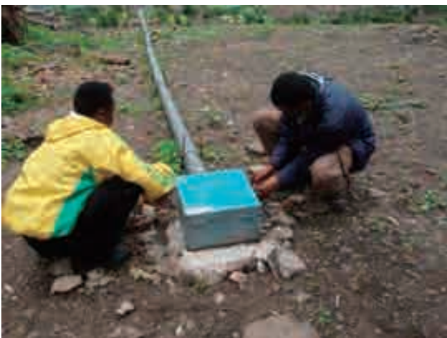
Installed extensometer at the landslide
