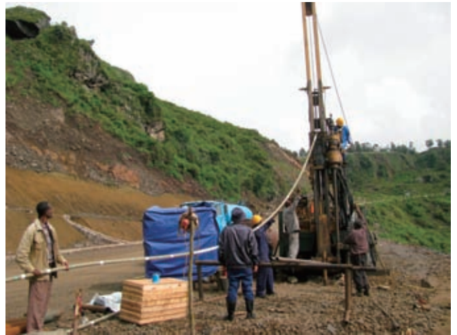
Drilling work at ST.0.800
