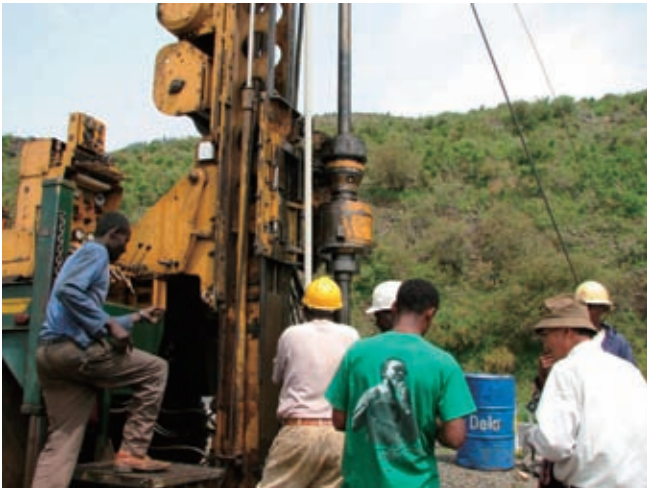
Technical transfer on drilling. Installation of casing pipes for inclinometer, 12 th Jul. 2011
