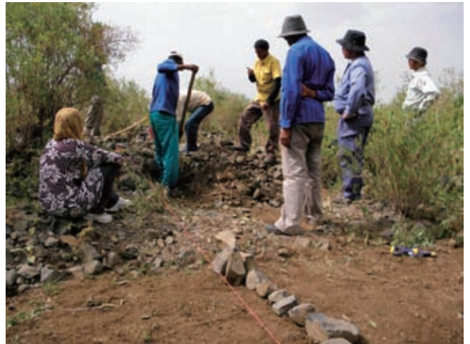
Digging trench for extensometer
