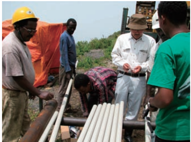
Technical transfer for connecting casing pipe for inclinometer, 13 th Jul. 2011
