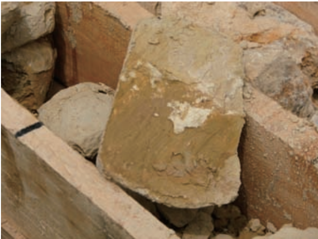
Slip surface on the core at B05-13
