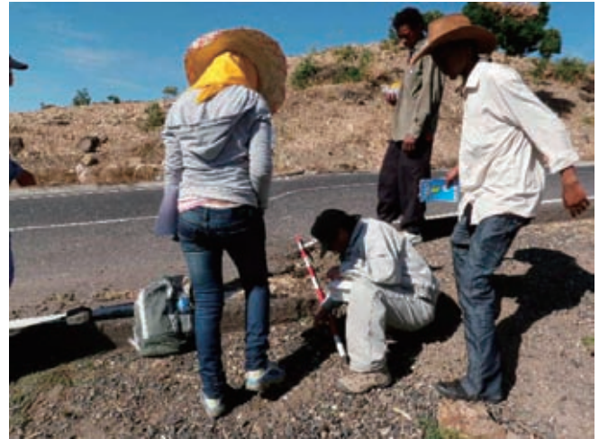
Technical transfer on site (Measurement method of cracks), 25 th Jan. 2011
