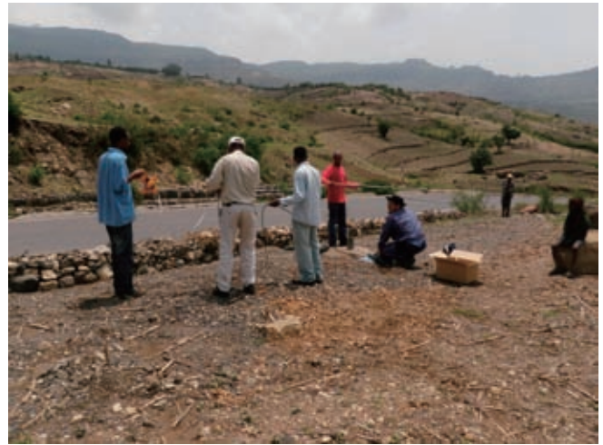
Installation of groundwater level meter, 22 nd Jun. 2011
