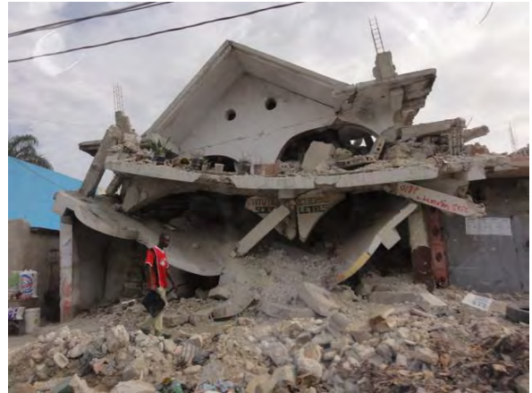
Photo 4: Wreckage of many collapsed houses still remained in Port-au-Prince. (July 2010)
