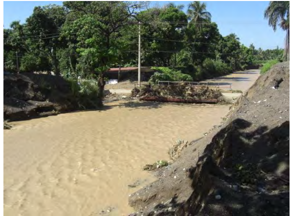
Photo 4: Former national road crossing overflowed Momance River after Hurricane Tomas (November 2010)
