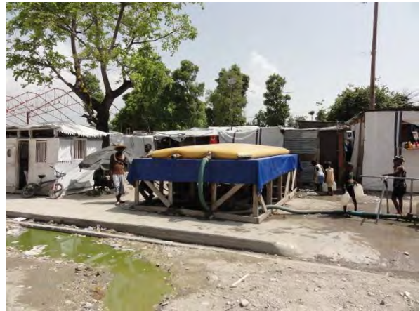
Photo 2: Bladders (plastic water tanks) installed in an evacuee camp and fed with water from a water truck (July 2010)
