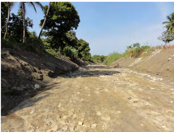
Photo 5: Sand from the upstream is chronically carried into and deposited on the bottom of Rouyonne River. Drastic measures are required. (January 2011)
