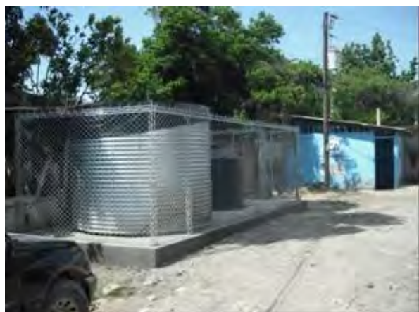
Water storage tank
