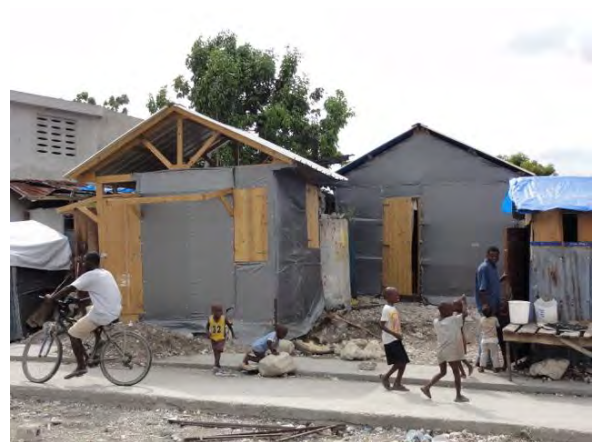
Photo 6: Temporary houses were gradually being built. (September 2010)
