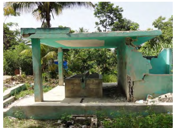
Photo 4: Public water tap in the suburbs of Léogâne, damaged and disabled by the earthquake (July 2010)
