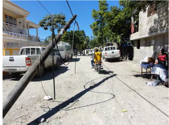
Photo 2: Electric poles fell over all over the commune. The transmission network is not functioning. (November 2010)
