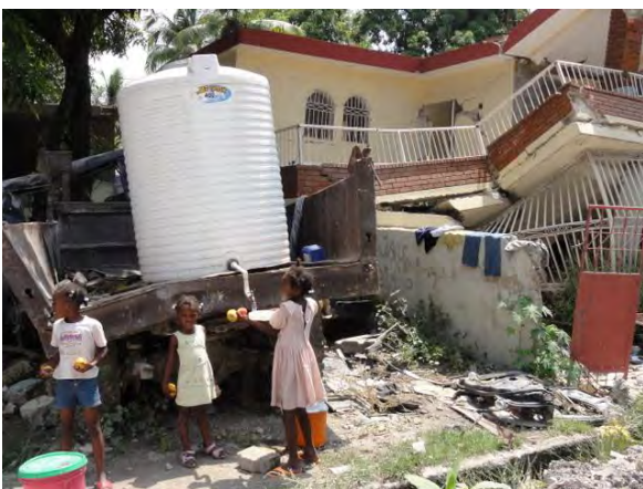
Photo 5: Children receiving water from a temporary feed tank in front of a collapsed house (July 2010)
