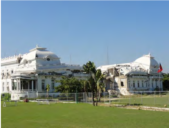
Photo 1: Collapsed Presidential Palace (November 2010)
