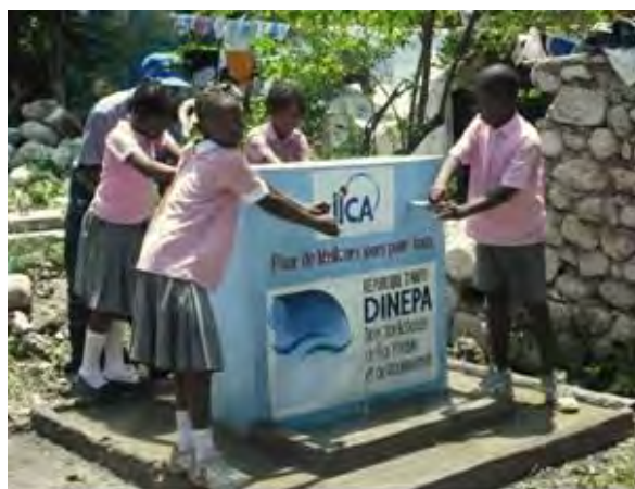
Public water tap at primary school
