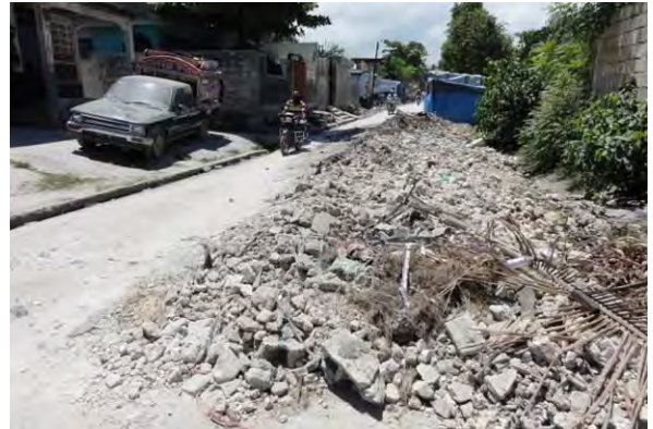
Photo 4: Wreckage left on a road in urban district (August 2010)
