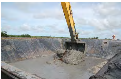
Excavated Soil in bucket on pontoon
