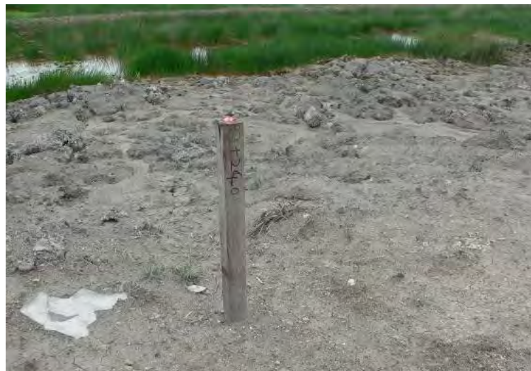
Picture 2.2.1 Slope of Embankment (Remained unrolled state)
