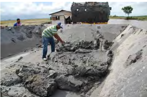
Cement adding and Mixing
