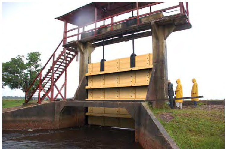
[ MADUNI RELIEF SLUICE DOOR in NEW FABRICATION ]
