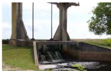
Notable Leakages
