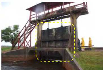
Existing Maduni Relief Sluice
