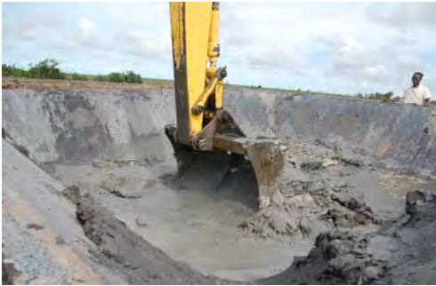
Cement adding and Mixing
