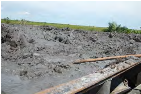
Excavated Soil stored in pontoon bucket at Field
