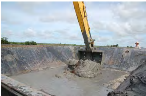
Excavated Soil in bucket on pontoon
