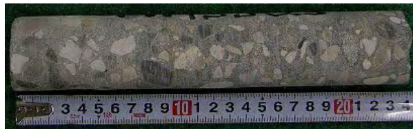
Figure 3.1.1 Core Sample in Local Section in the West Side (PW1SS0.5)
