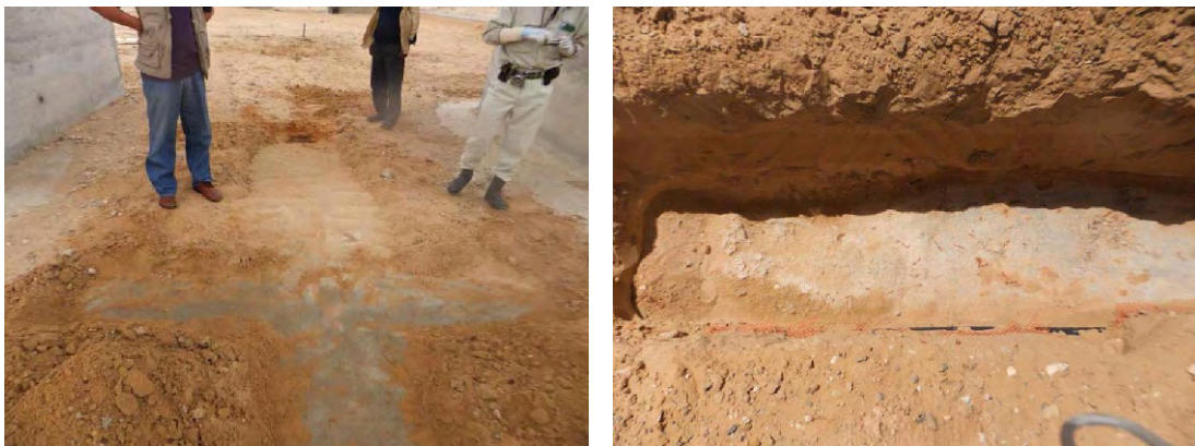
Photo 2.1.3 Upper Surface of Pile Cap in the East Side (Confirmed by Excavation)
