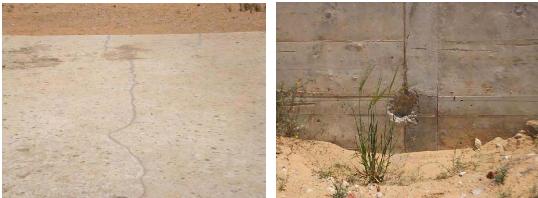
Photo 2.1.4 Crack on Pile Cap (Upper and Side Surface)
