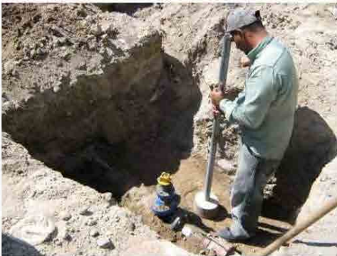
7. This is one of the valves they are starting to install.
