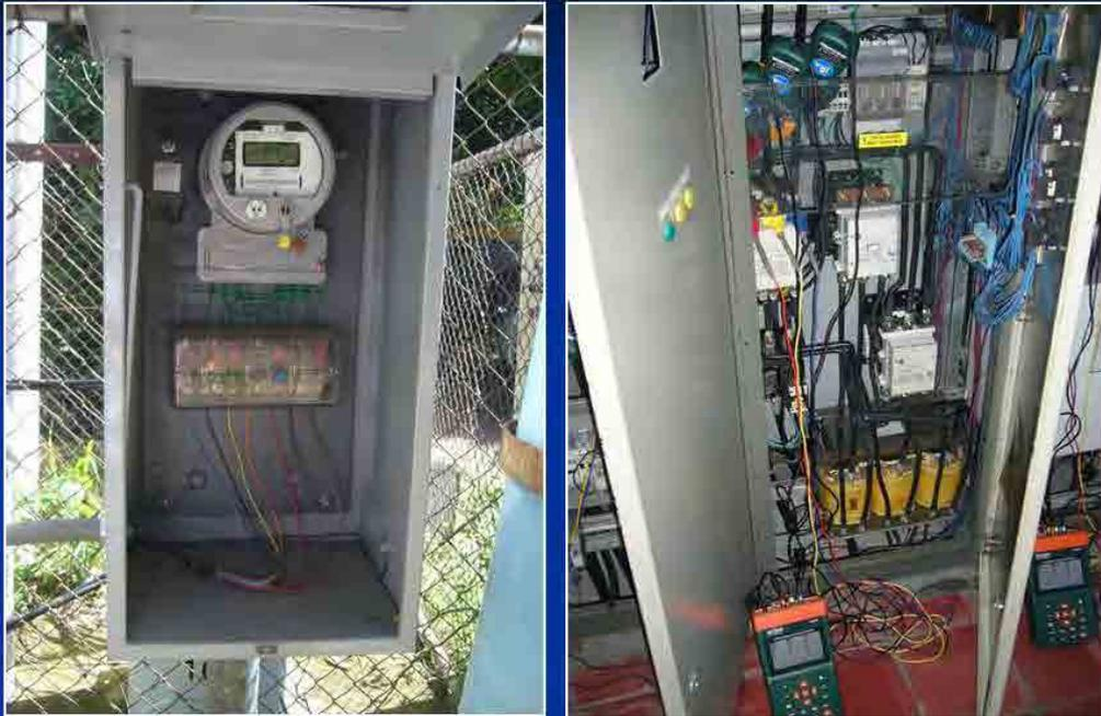
Fig.1 Watthour meter installed by CAESS or Power Analyzer 7
