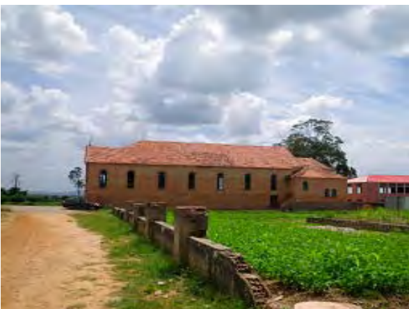
P3:Chicumbi Village Church (Low voltage distribution: 400-230V)
