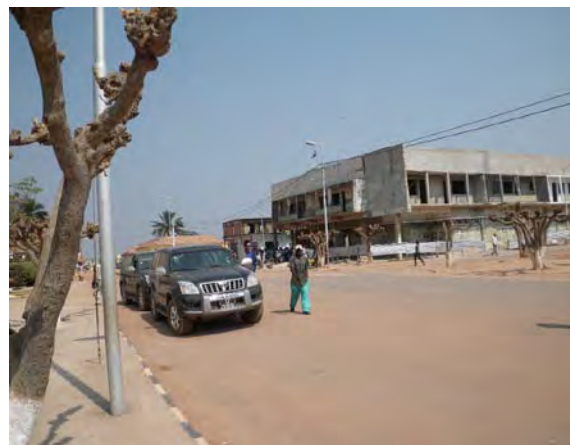
P4: Streetlights in Andulo city (230V)
