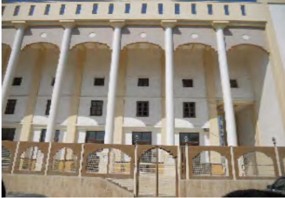
Picture 4.4-10 Insulation control by Canopy
