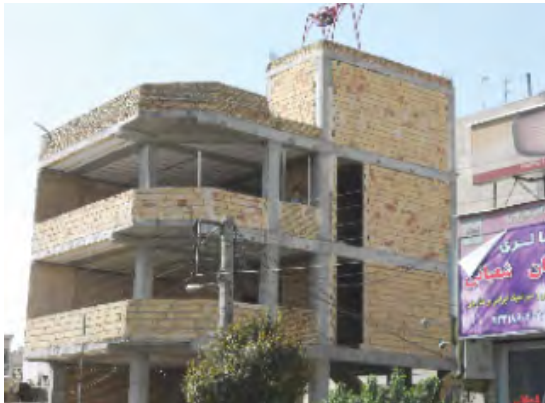
Picture 4.4-1 Example of Construction Method in Iran (hollow bricks filled into rigid concrete frame)
