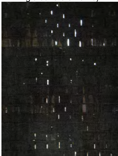
Picture 4.4-3 Look of Hollow Brick Wall in Execution from Inside (light leaks from the gap between bricks)
