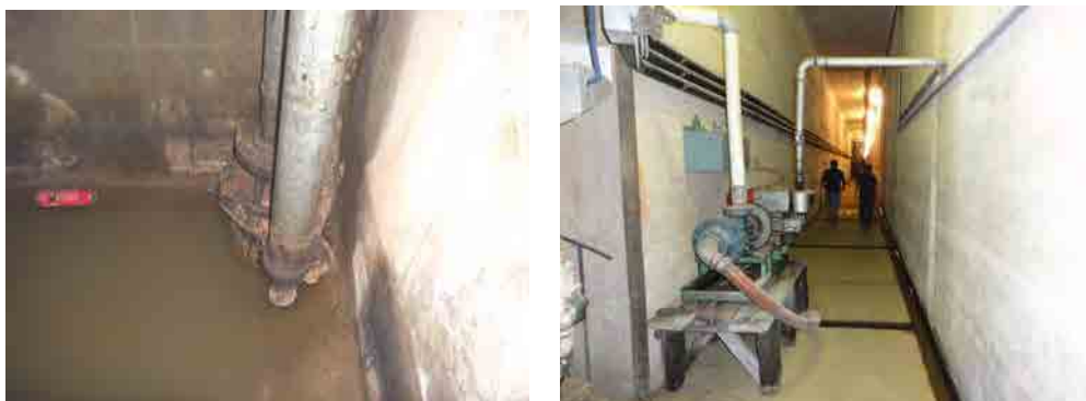
Drain pumps in Oeste Dam (left) and Sul dam (right)
