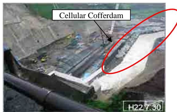
Figure 7.2.4 Example of Construction Cellular Cofferdam
