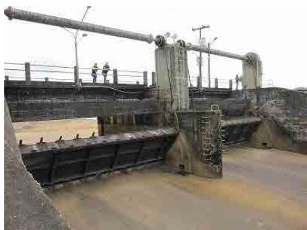
Spillway Gate (left) and Intake Tower (right) of Rio Bonito Dam
