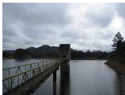
Spillway Gate (left) and Intake Tower (right) of Rio Bonito Dam
